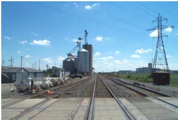
PHOTO 1: Looking east at Walnut Road crossing in New Carlisle, MP448.3 a proposed flyover location
