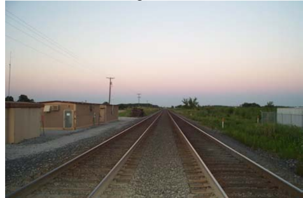
PHOTO 4: MP 364 at CR 47 looking east
