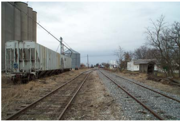
Photo 7: MP 78.7, at Center St. crossing in Woodburn, looking west
