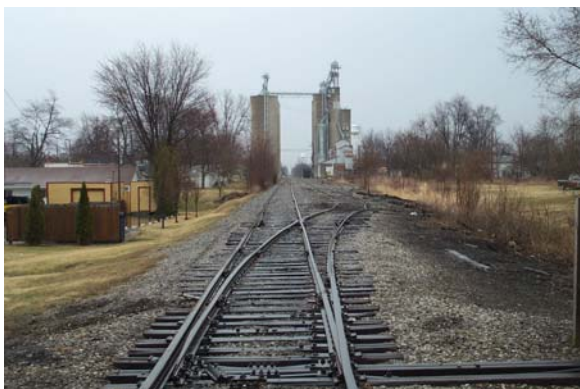
Photo 9: At Wentworth Rd. crossing near MP 72 in Antwerp looking east
