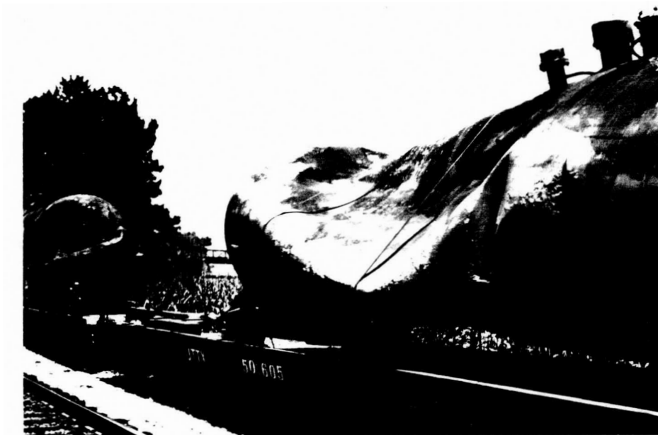
Photo C5-11: Crushed area of tank-car NATX 23367.
