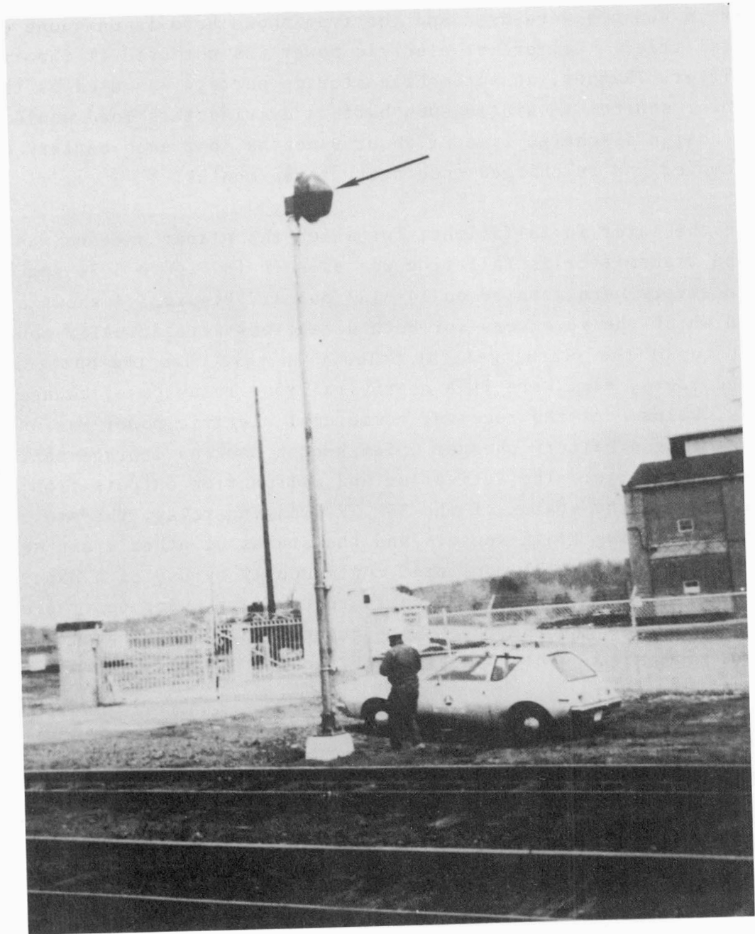
Figure 3.2 Receiver Installation - First Test Site
