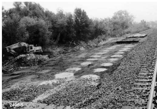
Figure 15 Stone columns installed in approach subgrade.
