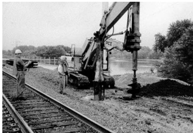
Figure 14 Hole boring in approach subgrade for stone column.
