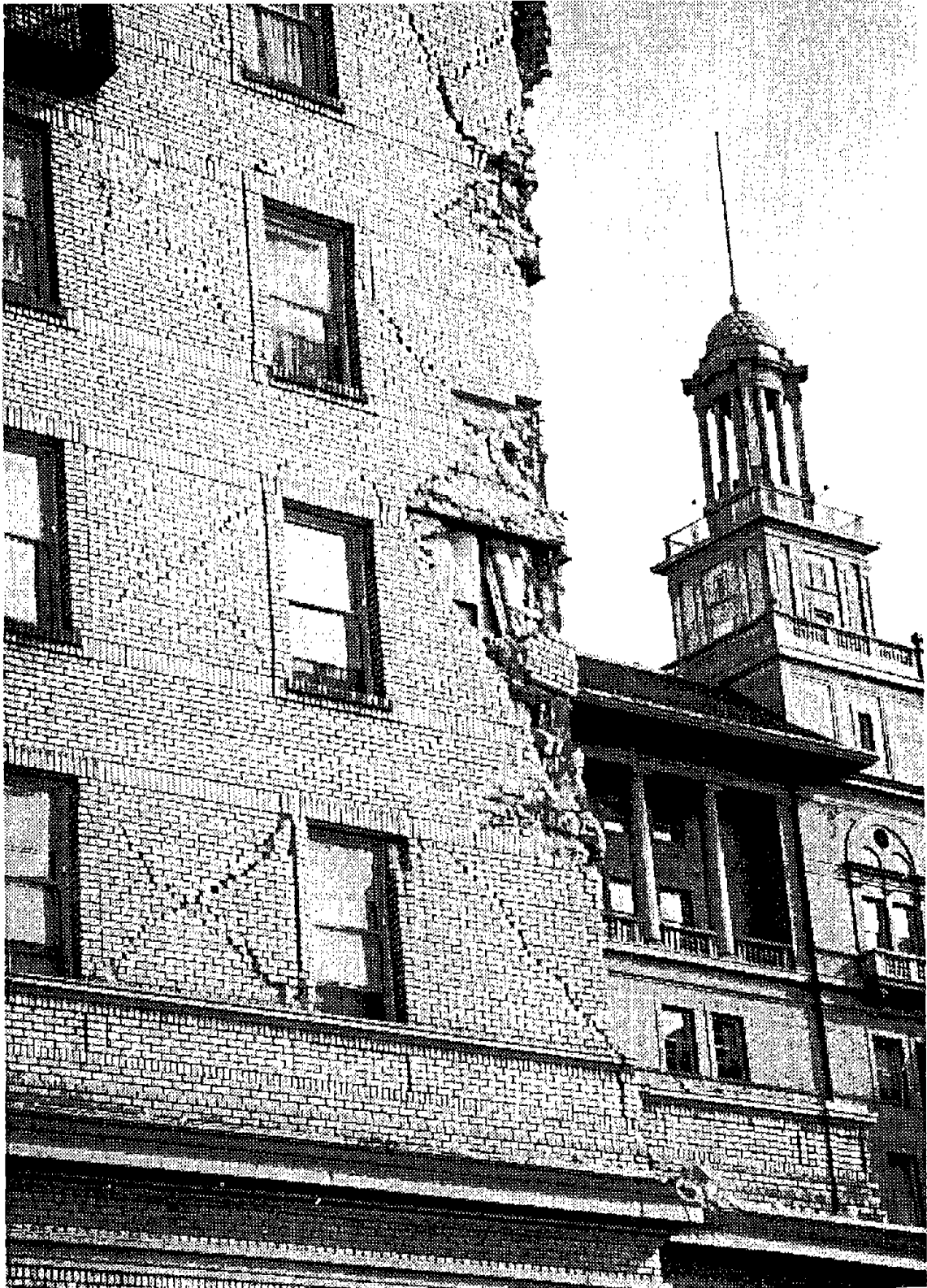
Figure B2-14 - Damage to Masonry Buildings in Oakland, Loma Prieta (1989)
