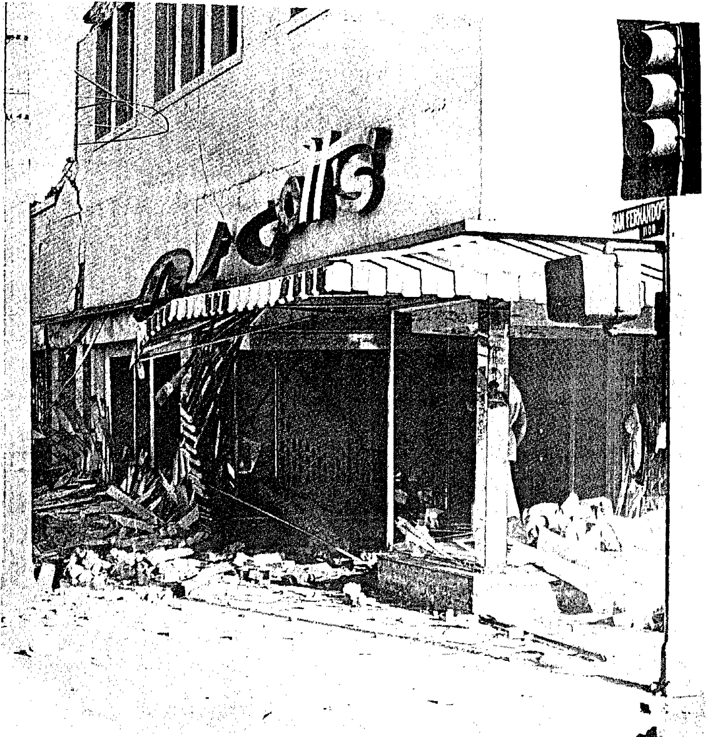
Figure B2-10 - Building Damage, City of San Fernando, San Fernando (1971)
