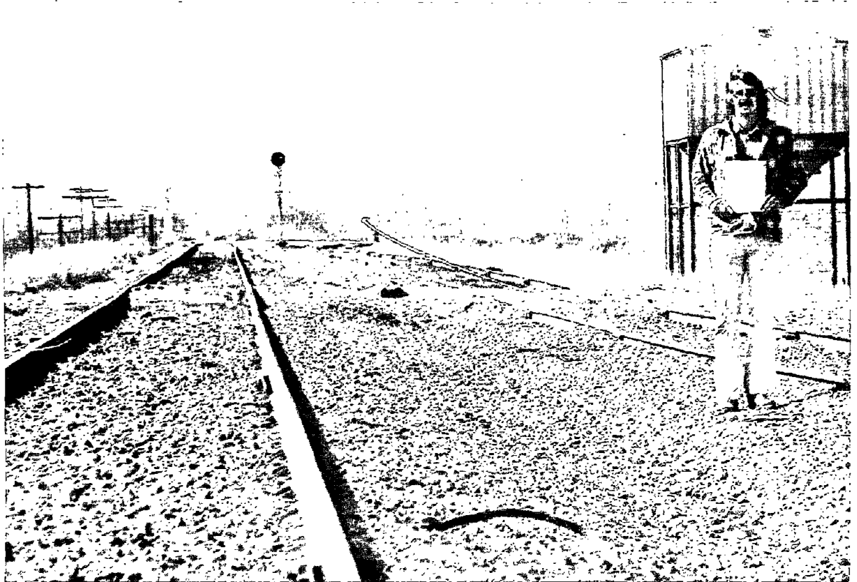
Fig. 3.1-4. Track roadbed at Heth.
