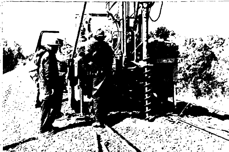
Fig. 2.3-2. Drilling in progress.
