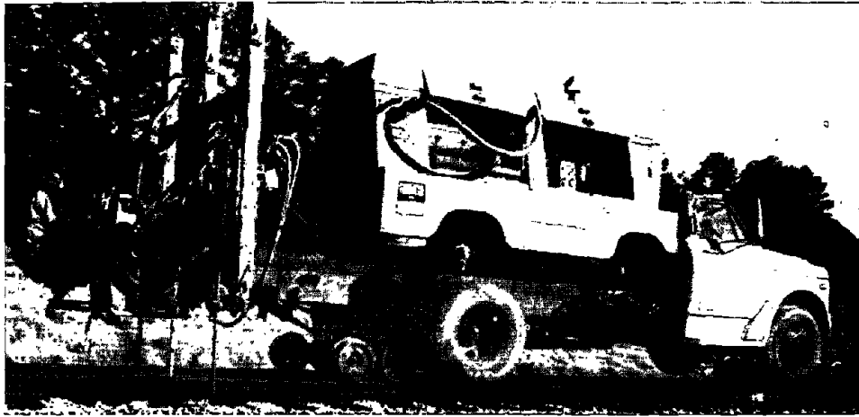
Fig. 2.2-5. Pneumatic drill truck.
