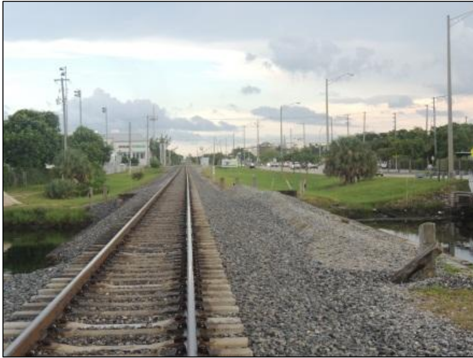
Figure 1-3.3 Bridge at MP 334.93
