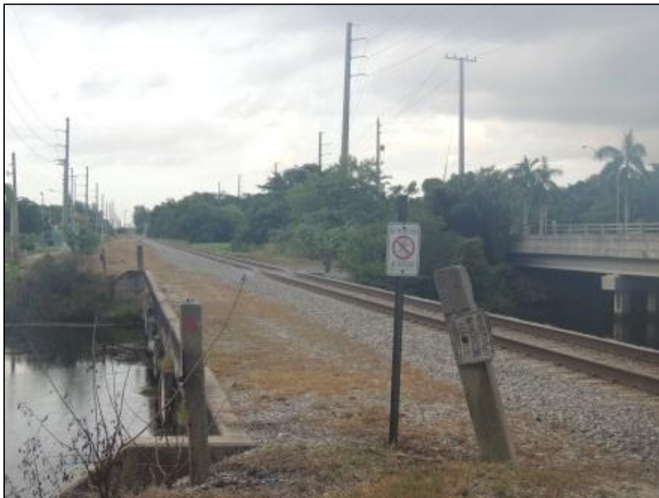
Figure 1-3.4 Bridge at MP 354.51
