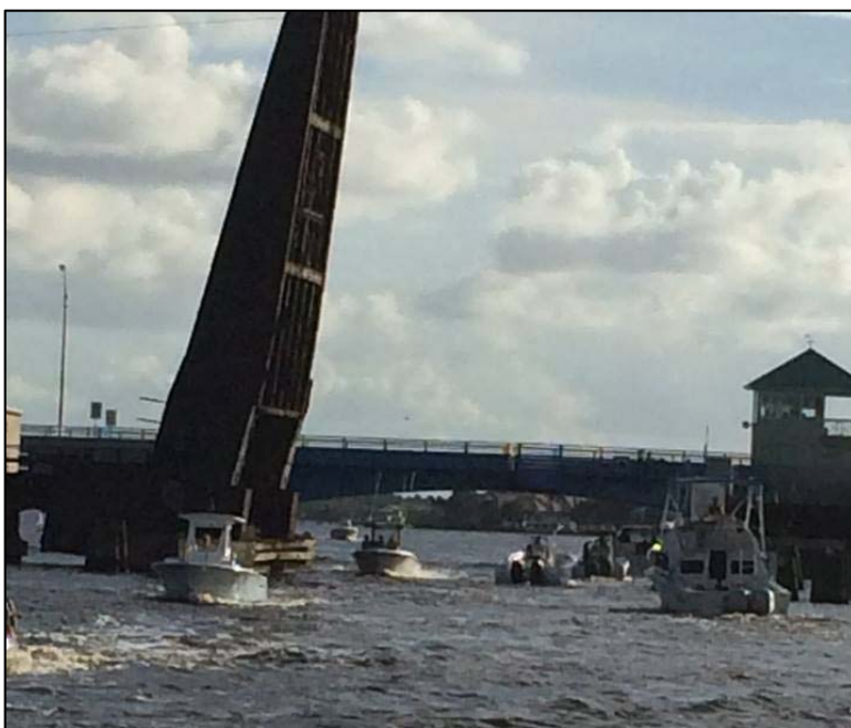
Figure 2-4. Boats crossing simultaneously in opposite directions (St. Lucie Bridge)
