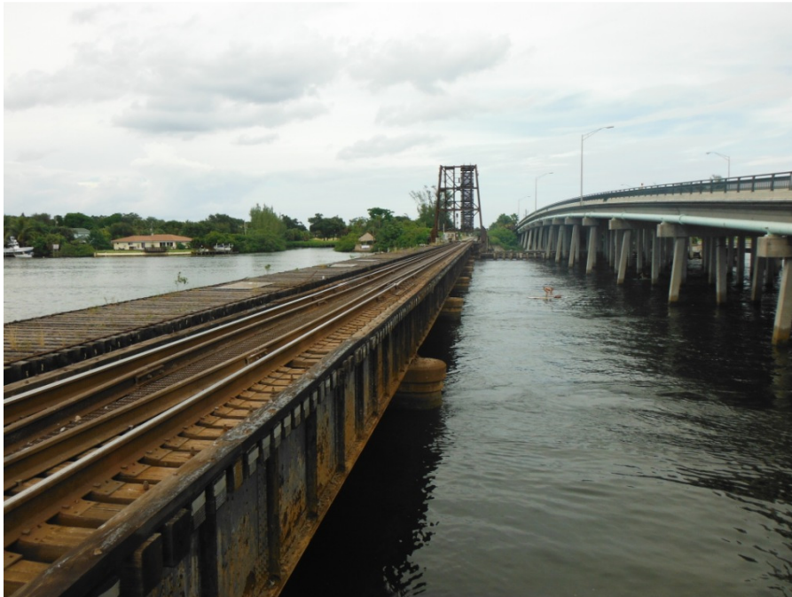
Photograph 13. Loxahatchee River Bridge (Mile Post 282.58), Facing north across the Loxahatchee River
