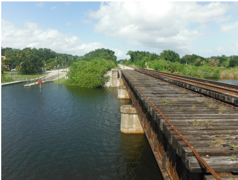
Photograph 6. Turkey Creek Bridge (Mile Post 170.70), View facing south
