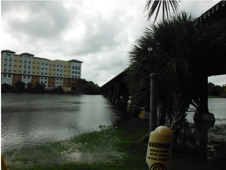
Photograph 3. Crane Creek Bridge (Mile Post: 194.47), Facing south from the northern bank
