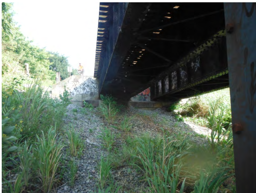
Photograph 8. Sebastian River (Mile Post: 212.07), South Side of the Sebastian River Railroad Bridge
