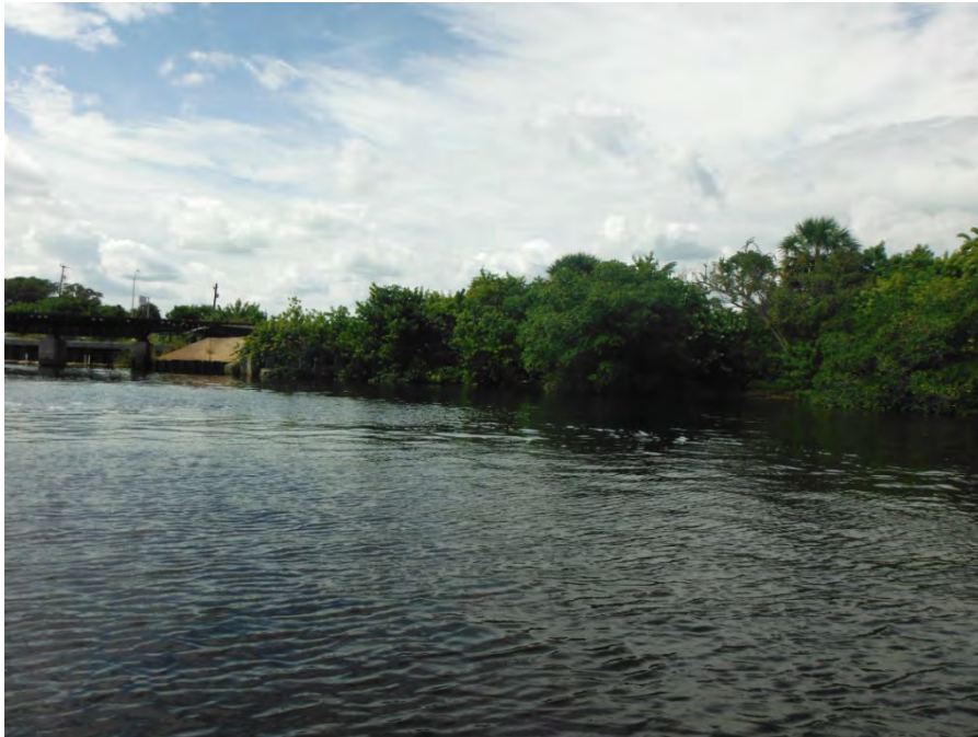
Photograph 11. St. Lucie River Bridge (Mile Post 260.93), Disturbed mangrove wetland located on the northern bank of the river
