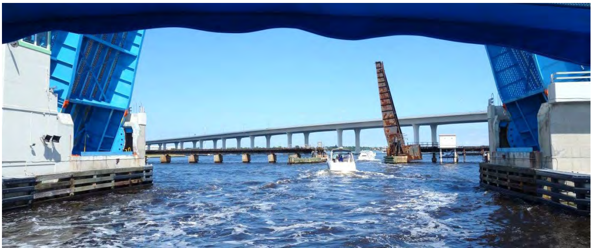
Single File Traffic Through St. Lucie River Railway Bridge
