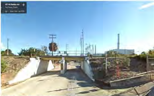
Figure 1: Avenue C Bridge
