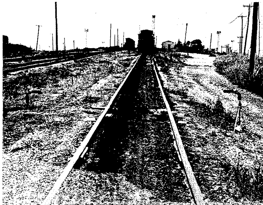
FIG. 6.5.4a VIEW OF THE EAST SIDE OF THE HUMP, INSPECTION PITS ARE INDICATED BY ARROW b VIEW OF THE MICROPHONES, EXCITERS AND WHEEL SENSORS
