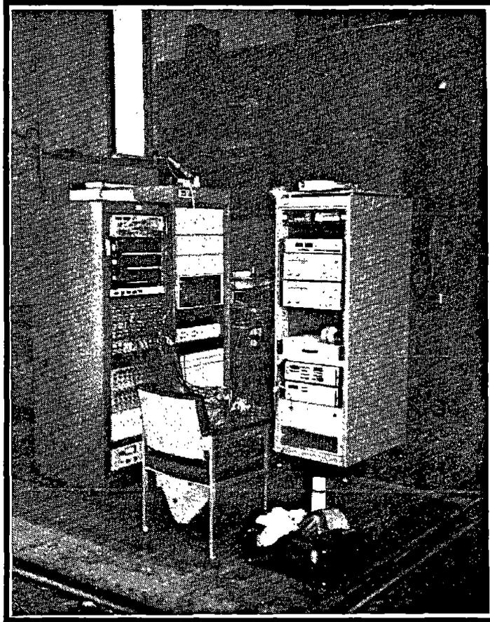
**Figure 8. Signal Conditioning and MTS Hydraulic Control System for MSU**
