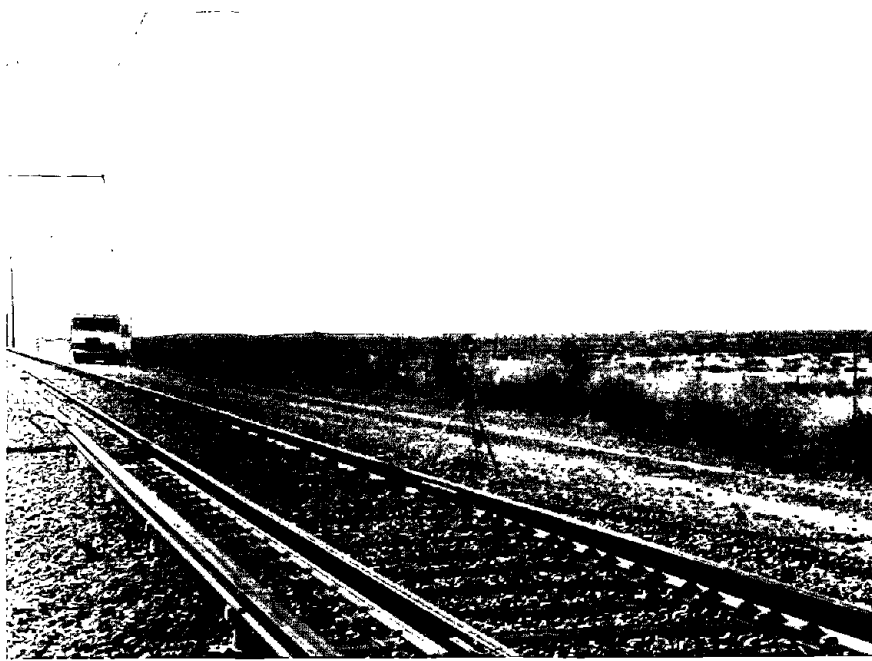
(a) Jointed Rail on Wood Ties.
