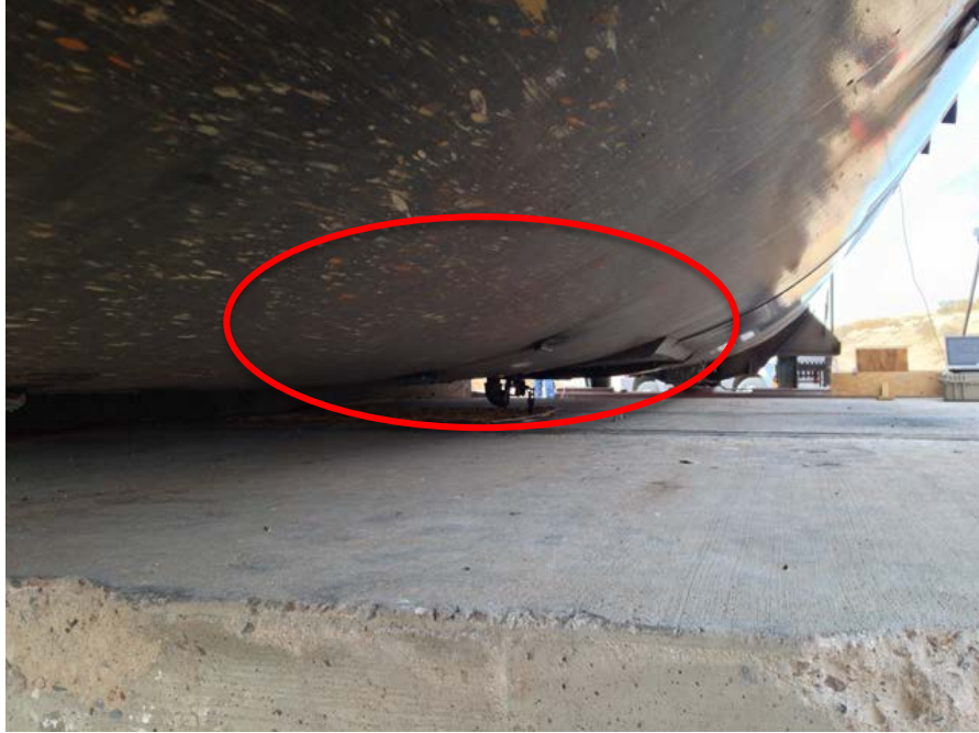
a) Localized jacket/tank transition
