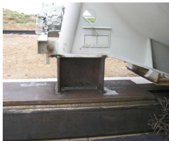
(b) Welded I-beam connection
