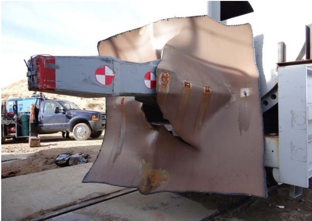
(b) Punctured tank shell
