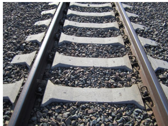
Figure 1. Half-frame ties installed in revenue service at the western mega site
