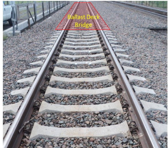
Figure 2. HFTs on the East Approach near Oshkosh, NE
