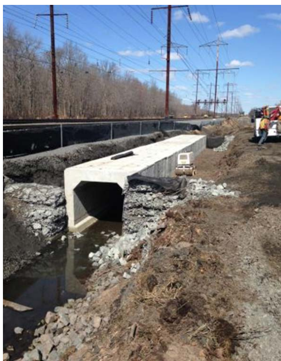
Track and Structure Upgrades
