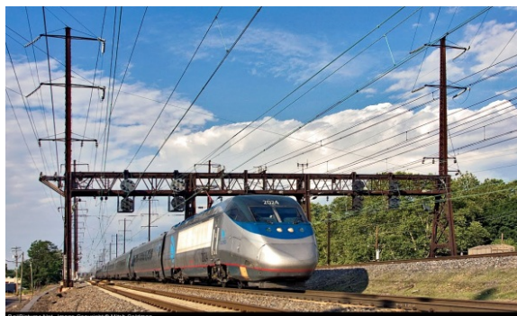
Traction Power Upgrades
