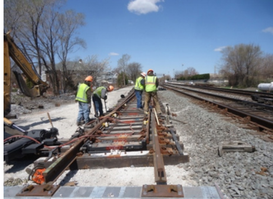
Contractors working on Turnout 9 (Hammond)
