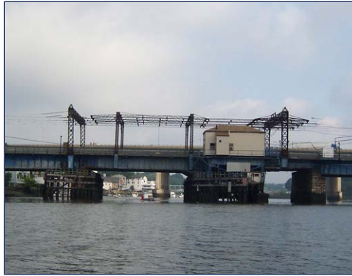
Saugatuck River Bridge (CT) 1904 $300M Replacement
