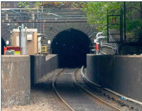
Hudson River Tunnels (NY/NJ) 1910 Multi-billion dollar Replacement
