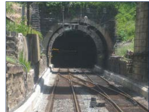
B&P Tunnel (MD) 1873 $1.5B Replacement
