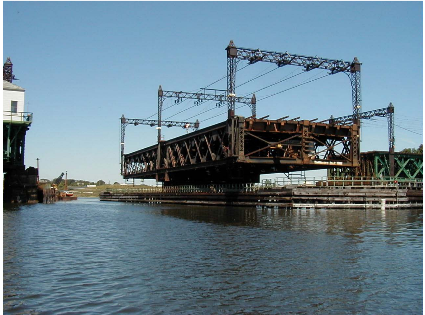
Norwalk River Bridge, CT
