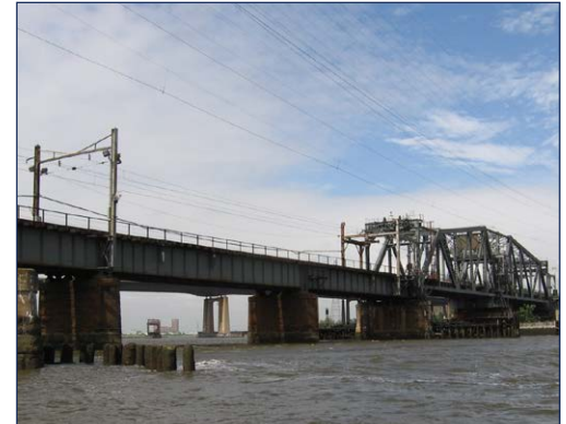
Portal Bridge (NJ) 1906 $1B Replacement
