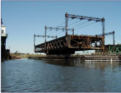
Norwalk River Bridge (CT) 1896 $250M Replacement
