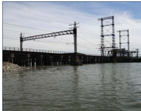
Pelham Bay Bridge (NY) 1907 $250M Replacement
