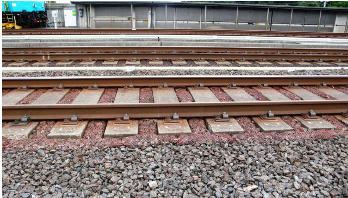
Figure 3.4: Ballast bags placed on the Japanese Shinkansen
