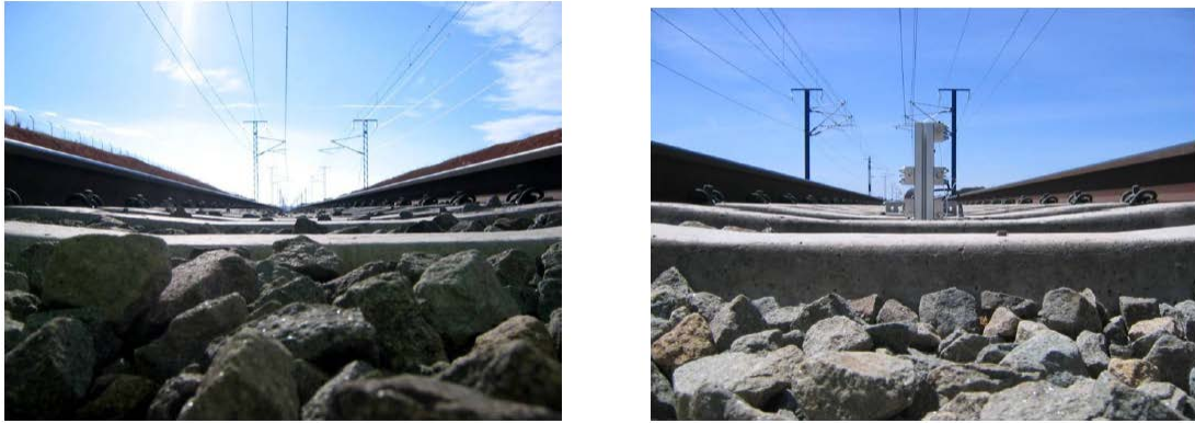
Figure 3.3: The effect of lowered ballast profile: ballast particles may be less exposed to ballast motion.
