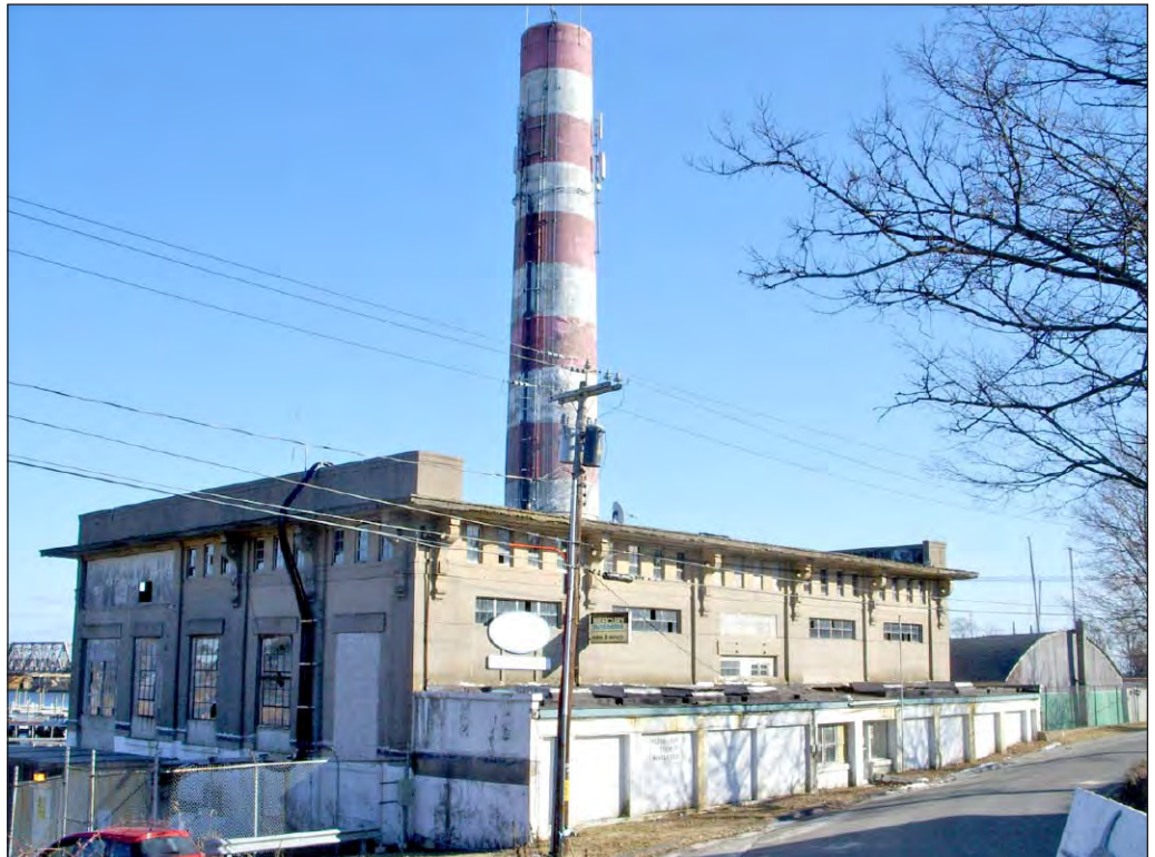
The north and west facades of the building at 2-20 Clark Street. Note the single-story addition appended to the west façade. While most of the clerestory windows remain intact, many of the larger windows along the facades have been truncated or sealed.
