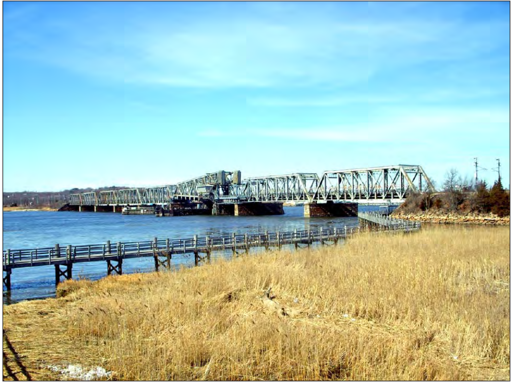
The Connecticut River Bridge, which carries Amtrak's Northeast Corridor over the Connecticut River, as seen from the Ferry Landing Park in Old Lyme, looking northwest.
