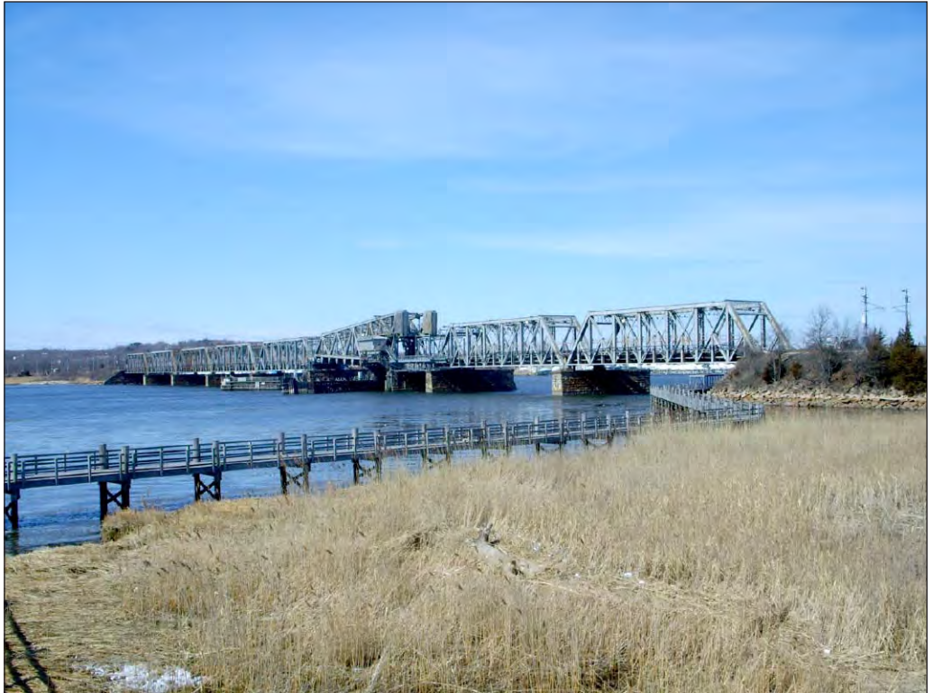
Looking northwest from Ferry Landing Park in Old Lyme, a view of the Connecticut River Bridge, which carries Amtrak's Northeast Corridor across the Connecticut River. The bridge is listed on the State Register of Historic Places (SR) and has been determined eligible for the National Register of Historic Places (NR) as part of the Moveable Railroad Bridges on the Northeast Corridor in Connecticut Thematic Resource. 1
