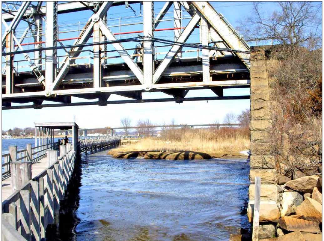
Looking north from the wood walkway in the Ferry Landing Park in Old Lyme, immediately south of the Connecticut River Railroad Bridge. The Baldwin Bridge, which carries I-95 and the Boston Post Road over the Connecticut River, is pictured in the background.
