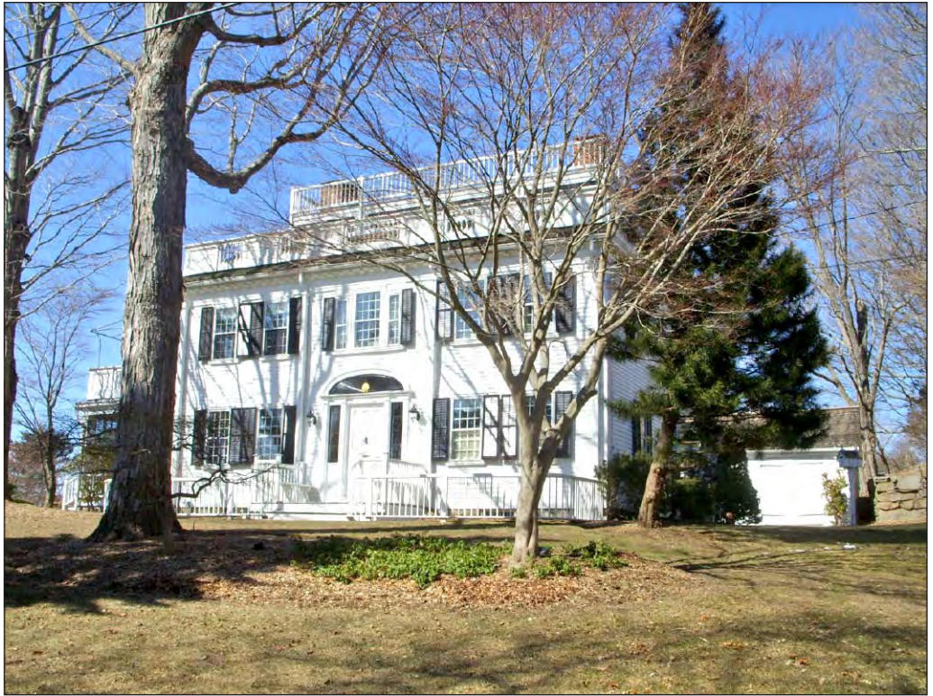
The front (south) façade of the Enoch Noyes House (the “House on the Hill”), located at 317 Ferry Road in Old Lyme, roughly a quarter of a mile north of the project site. The ca. 1820 Federal-style house is clad in wood clapboard and has brick side chimneys
