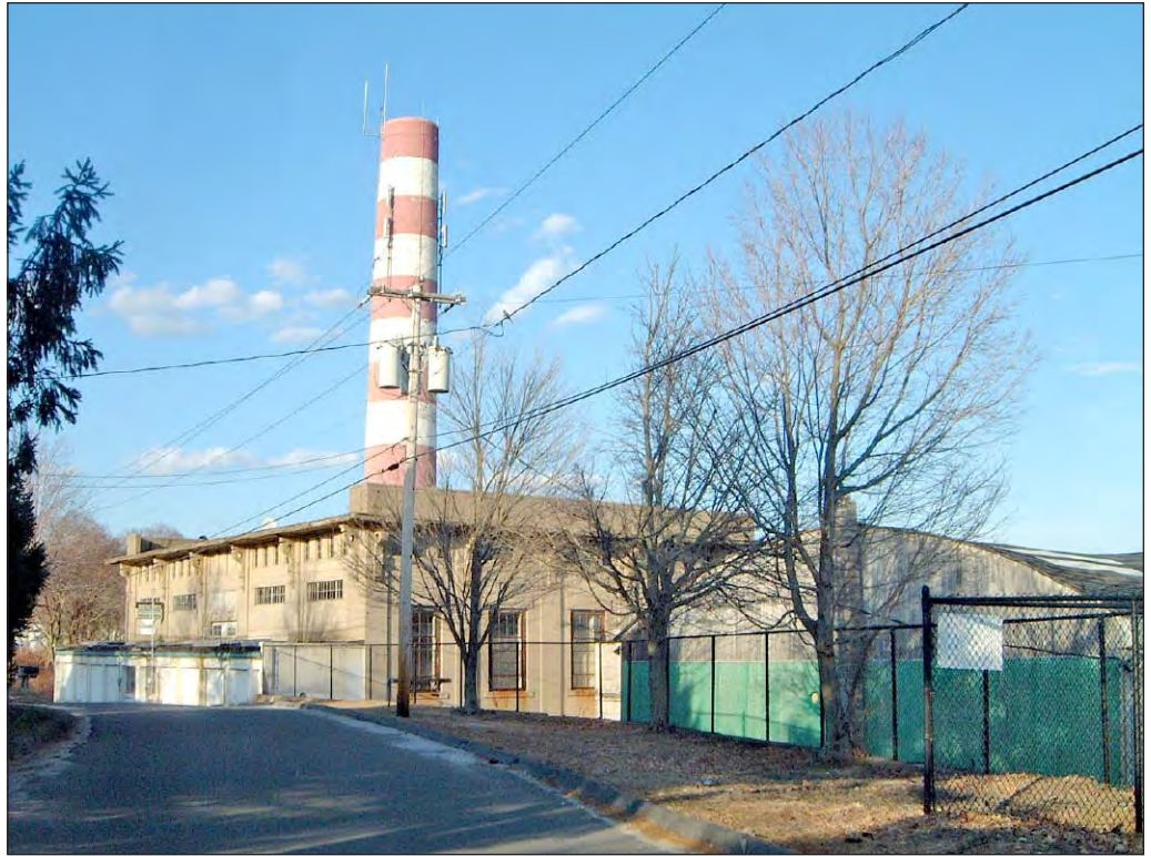
The west and south facades of the building at 2-20 Clark Street, viewed from the southern portion of Clark Street in Old Saybrook. The parged masonry structure has decorative eaves brackets, large metal windows and simple pilasters. A single-story addition has been appended to the west façade (left); and a large corrugated metal structure has been connected to the south façade (right).
