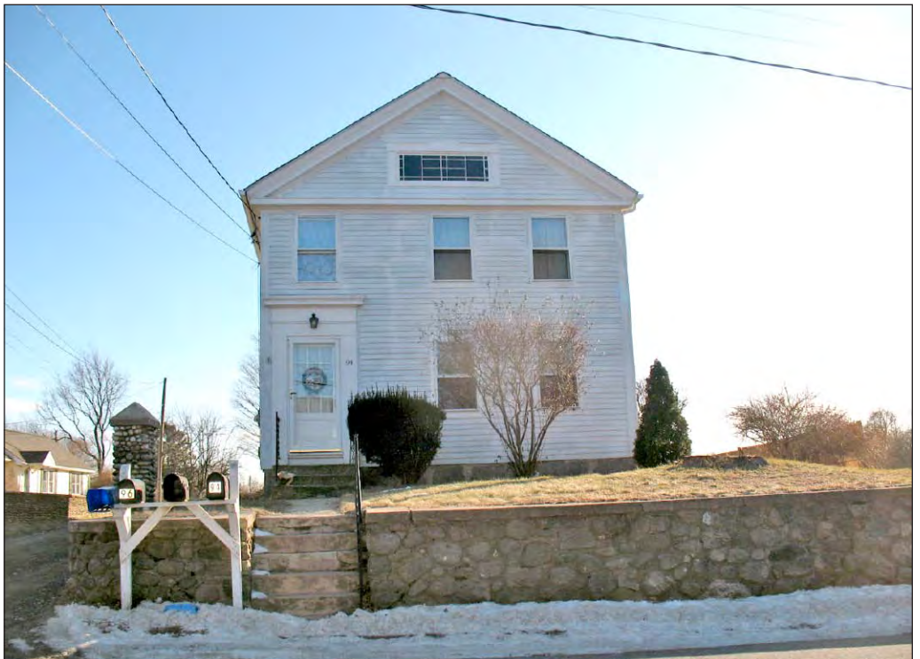
The house at 94 Ferry Road in Old Saybrook, roughly 500 feet north of the project site, is a late Federal-style house with a raking cornice, classical door frame, and a decorative gable window. It is clad in wood clapboard. Most of the windows have been replaced with modern sash.
