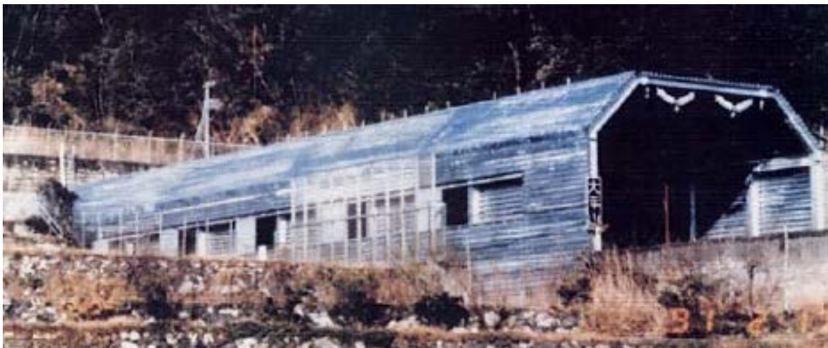
Figure 63. Japanese tunnel entrance hood (steel) – retro-fitted to Ohirayama tunnel, from Maeda et al [226]
