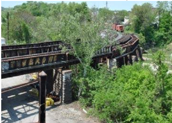
Image 10: Baltimore and Ohio Belt Line Bridge over Jones Falls Valley
