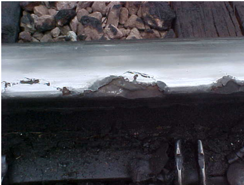
Figure 48: Gauge Side Shell Showing Severe Parent Metal Decay
