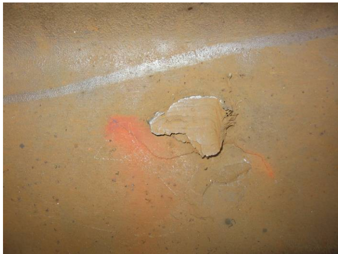
Figure 42: Web Defect Developing from Bond Application
