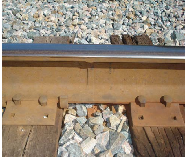
Figure 54: Electric Flash Butt Weld in Track
