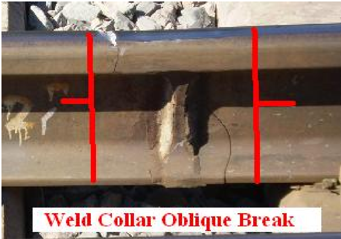
Figure 39: Thermite Weld Showing Oblique Type Failure Originating in Web Area
