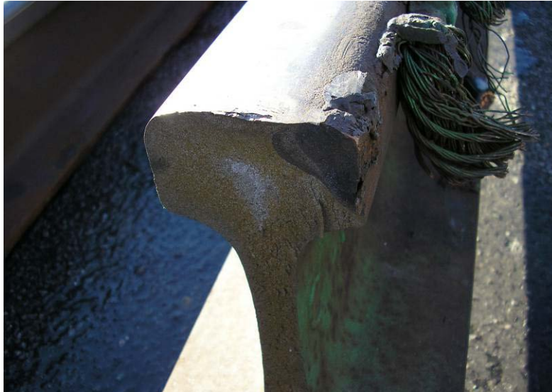
Figure 41: Transverse Defect Developing from Bond Application
