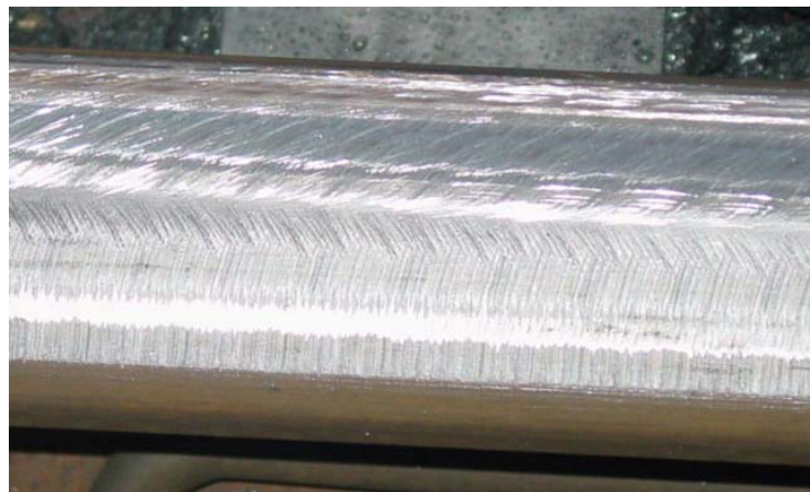
Figure 59: Freshly Ground Rail
