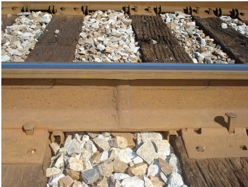
Figure 56: Gas Pressure Weld in Track
