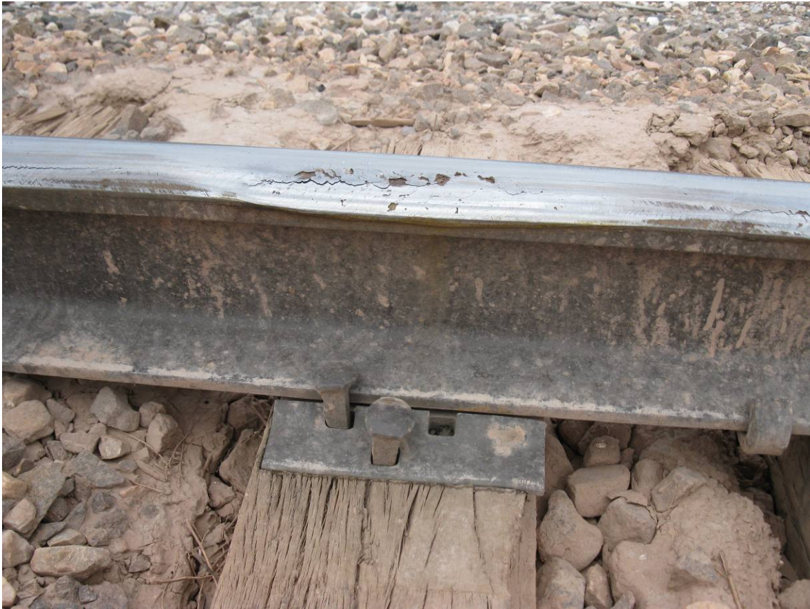
Figure 44: Flattened Rail
