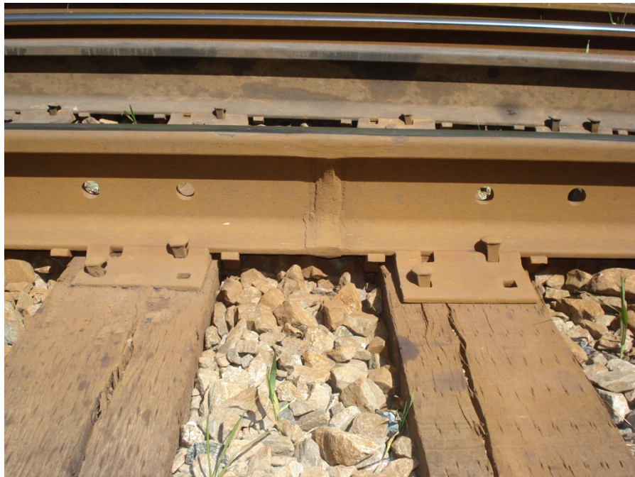
Figure 57: Thermite Weld in Track
