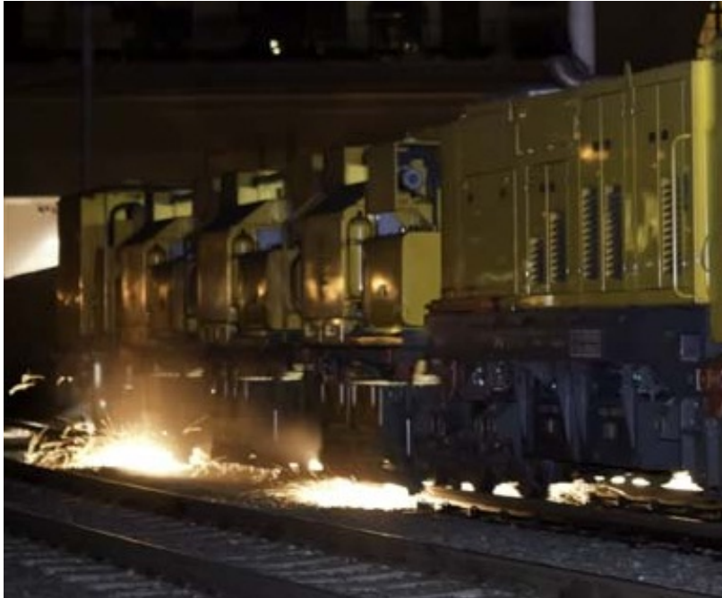
Figure 60: Rail Grinder at Work
