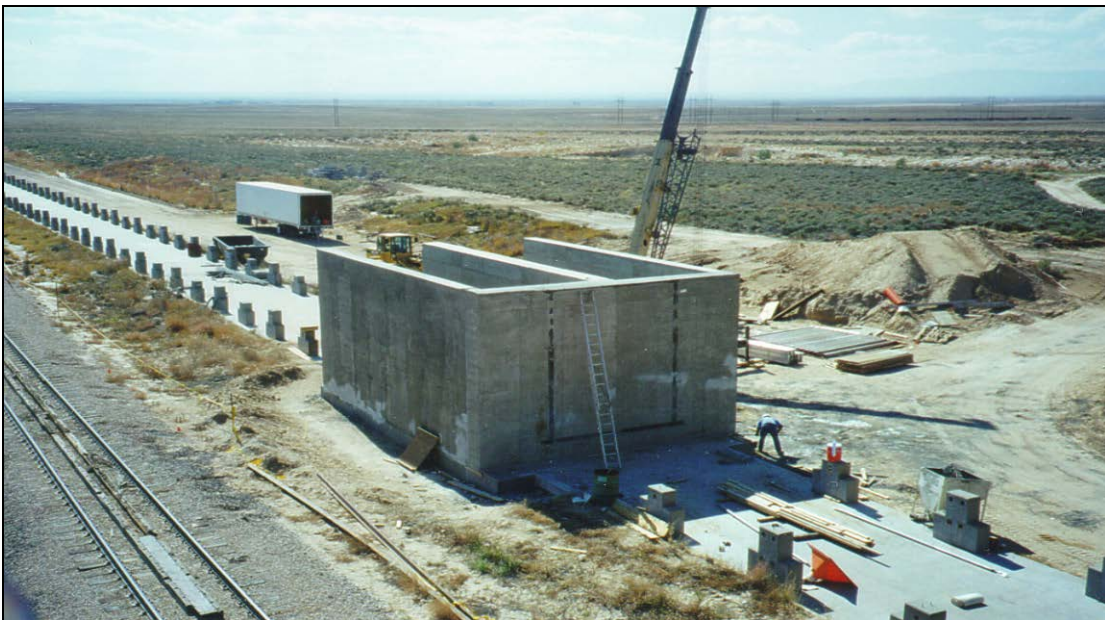
Figure 46. Vehicle Impact Wall Under Construction
