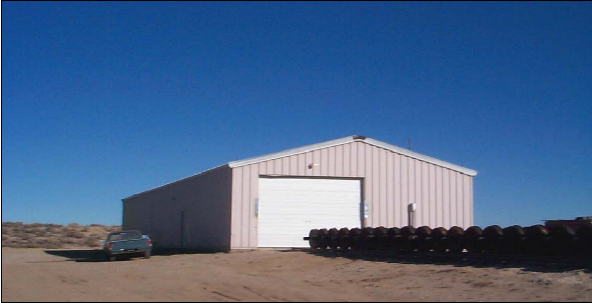
Figure 21. The LIMRV Maintenance Building
