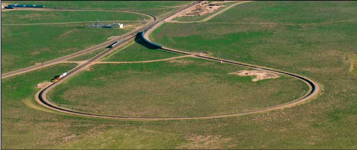
Figure 30. Balloon Loop Looking Northwest
