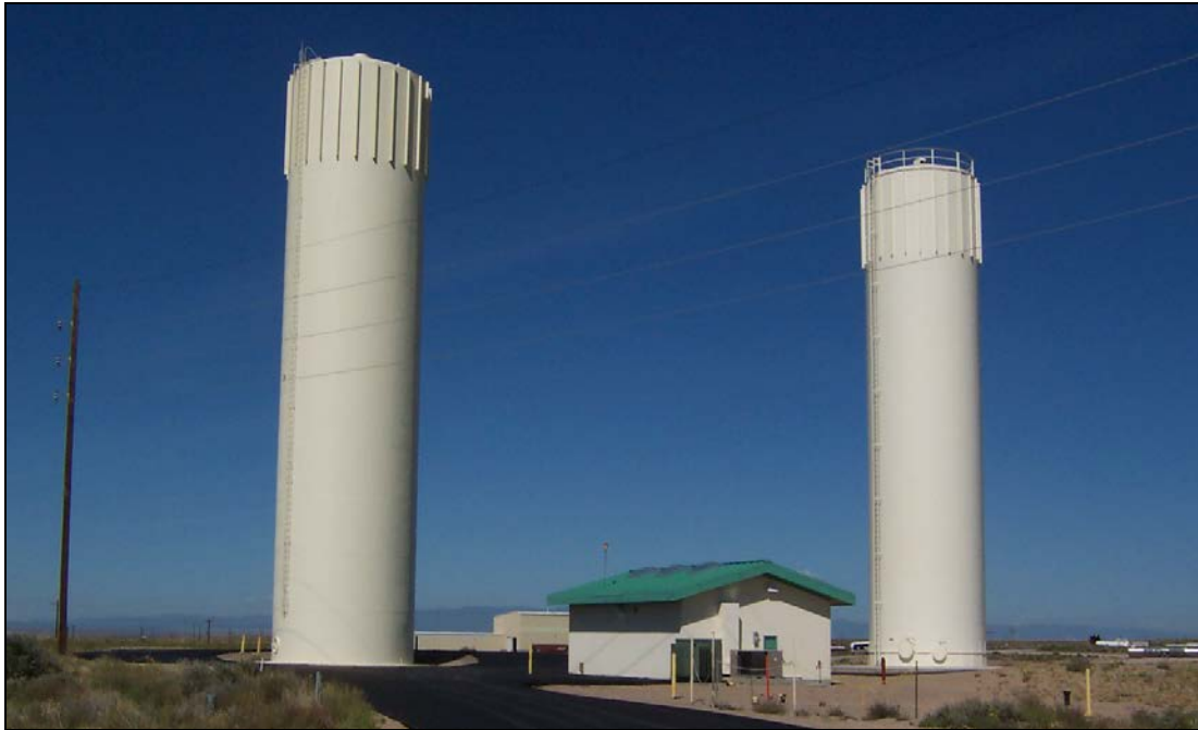
Figure 50. Water Reservoir and Distribution Pump House.
