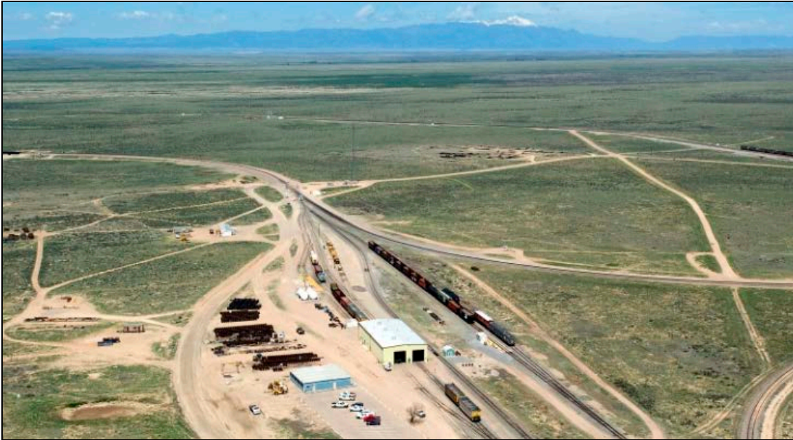
Figure 18. The FAST Modular Building (left) and the FAST Maintenance Building (right)
