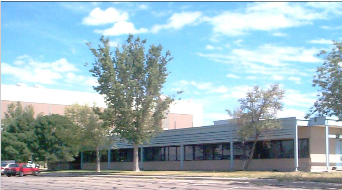
Figure 6. The Project Management Building (PMB)
