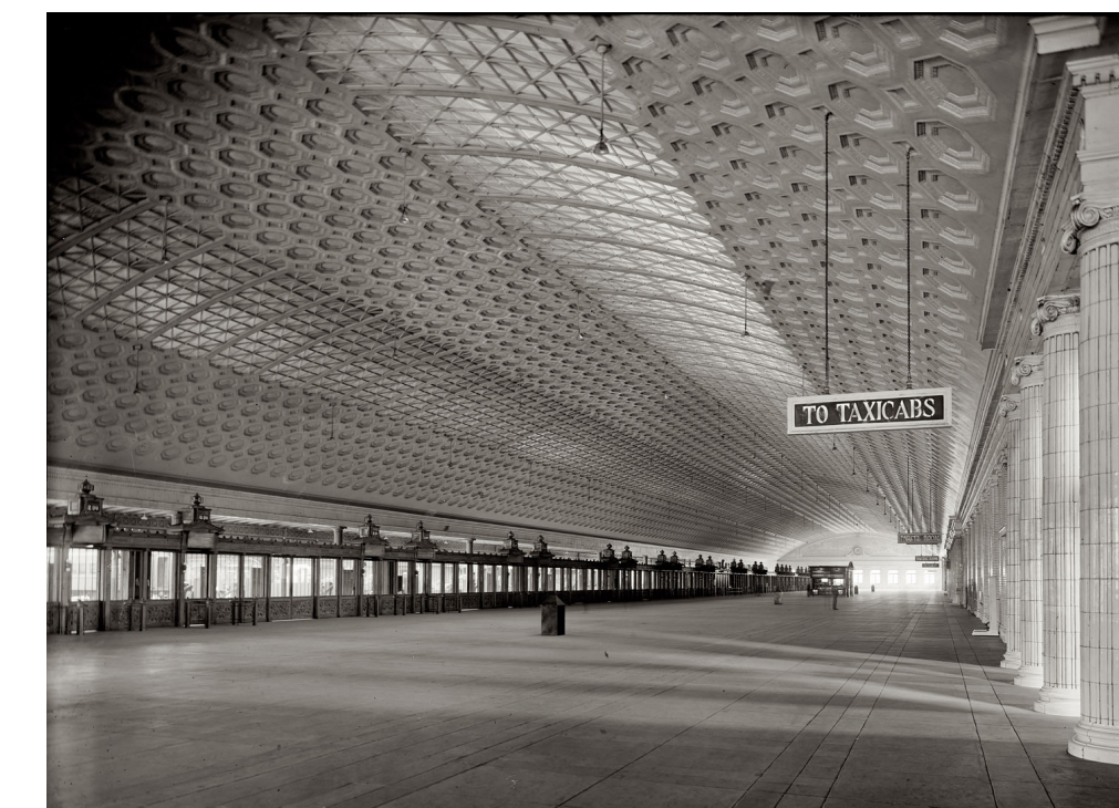
Union Station – Historic Concourse Washington, DC
