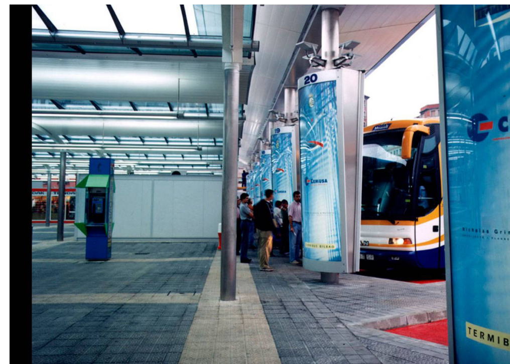
Bilbao Bus Terminal Bilbao, Spain
