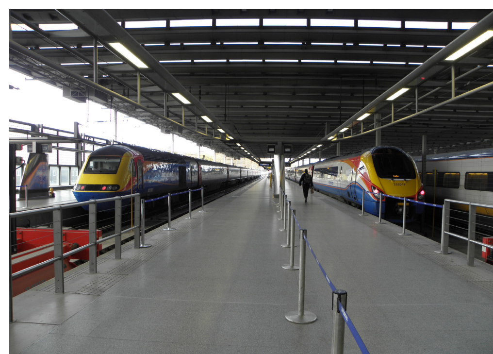
St. Pancras Station London, England
