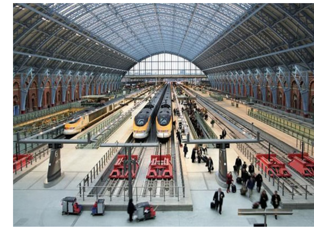
St. Pancras Station London, England
