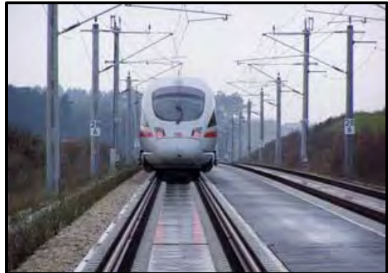
Typical Overhead Catenary
