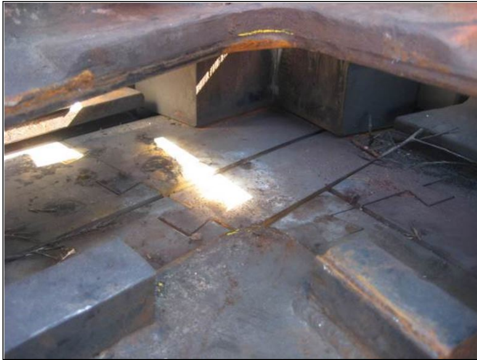
Figure 94. Nortrak pad material in good condition after 35 MGT
