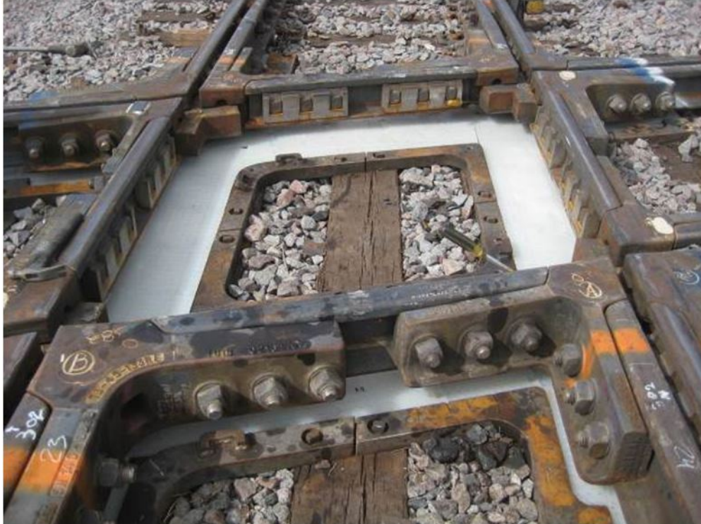
Figure 11. Nortrak-designed pad in place between the milled platework and the castings. View with the center guardrail piece removed.
