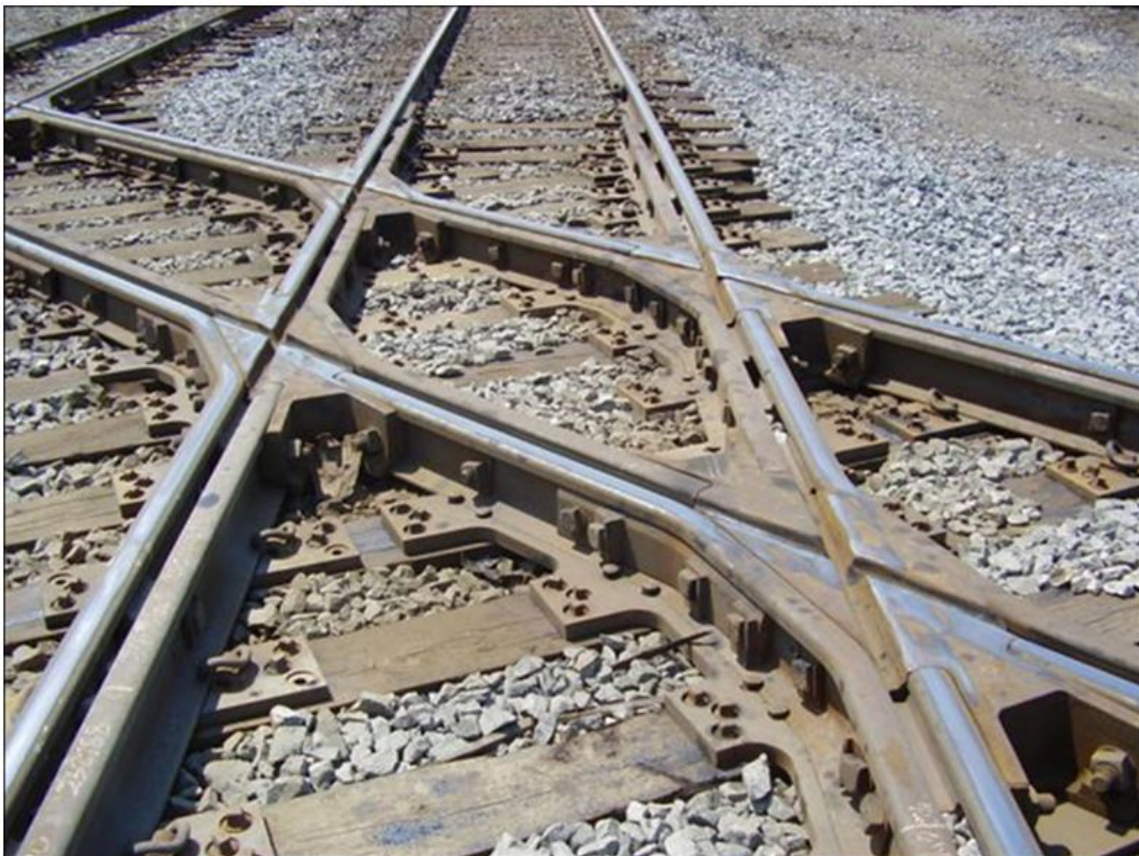
Figure 1. An Intermediate Angle Cast Crossing in Revenue Service
