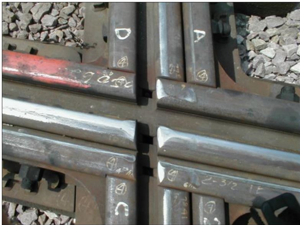
Figure 3. Three-Rail Crossing Diamond
