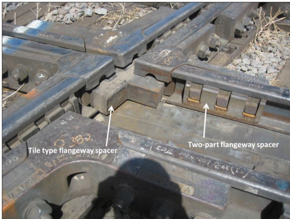
Figure 7. Tile type flangeway spacer at the casting corners and two-part (split) running rail/guardrail flangeway spacer
