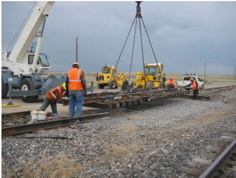
Figure 9. Test prototype crossing diamond installation
