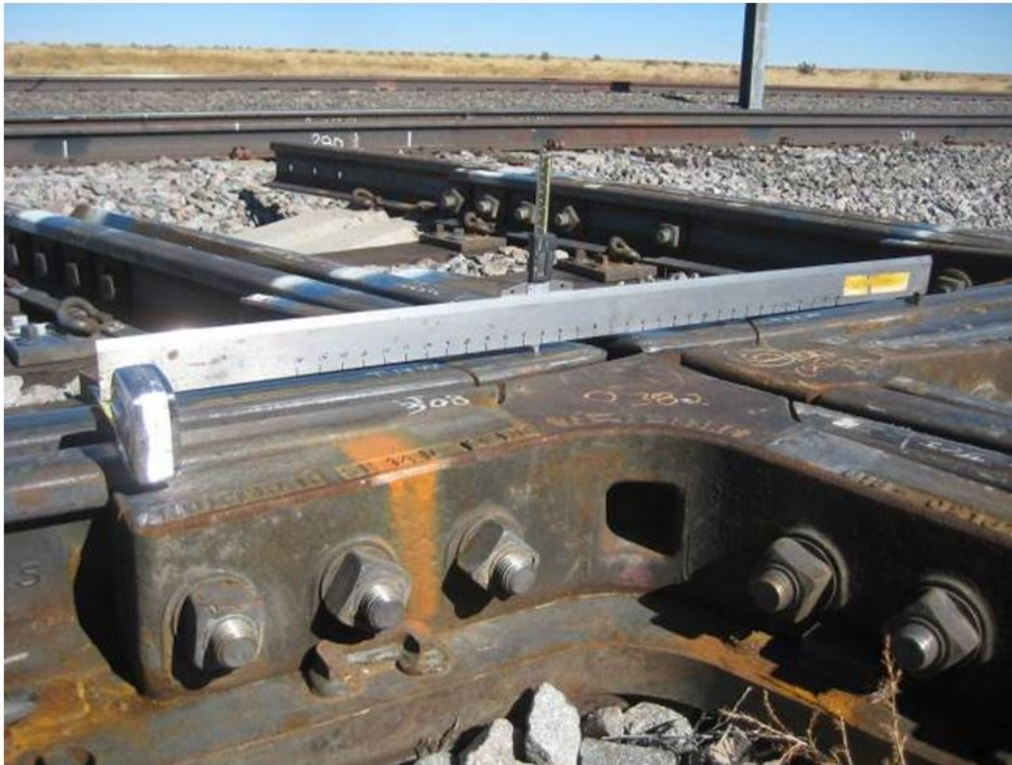
Figure 32. Longitudinal profile measurements at 1-in intervals across the casting corners using a steel straightedge and digital depth gage
