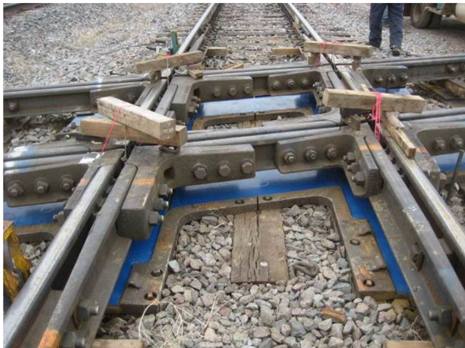
Figure 18. Getzner Type B full-coverage rail seat pad in place
