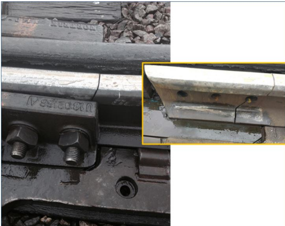
Figure 102. The leg rail on the northwest frog broke after 59 MGT
