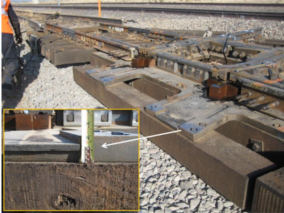
Figure 8. Milled platework and 0.5-in rubber pads
