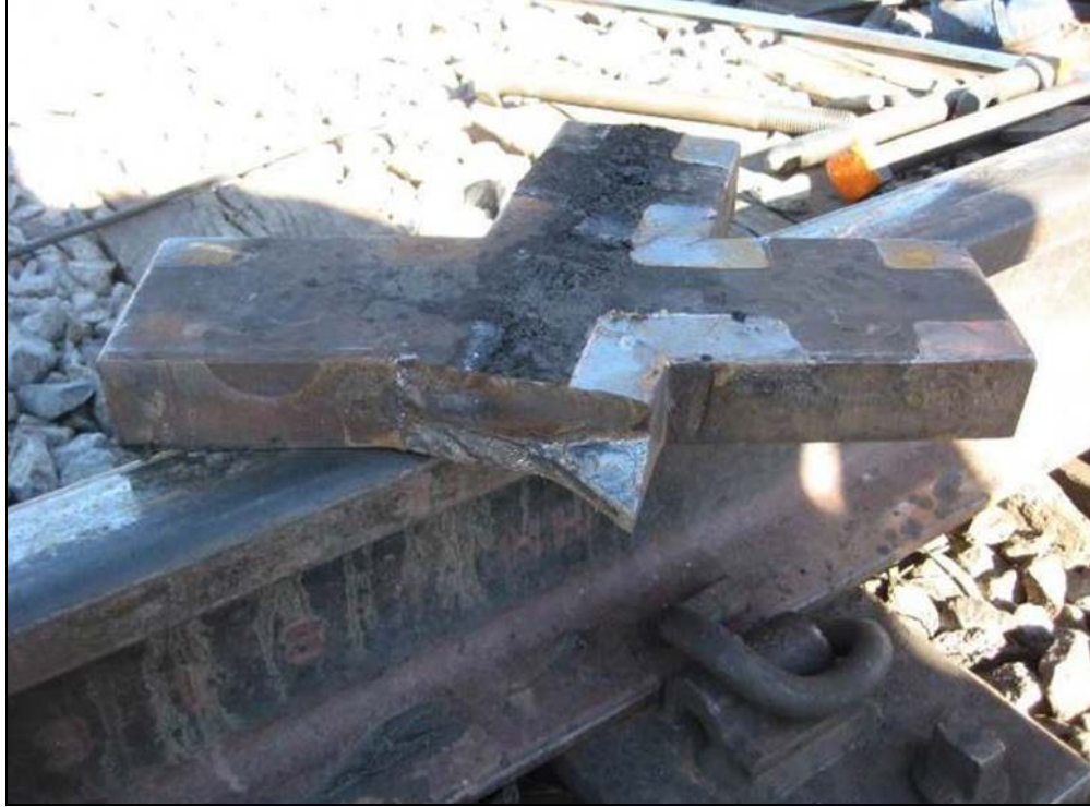
Figure 105. The top half of a layered flangeway spacer tile broke and was replaced
