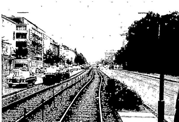
P-52. Staggered stops in a median to minimize ROW width (Cologne)
