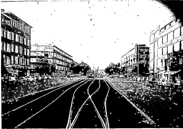
P-36. A third track permits overtaking of a car waiting for left turn (Rotterdam)
