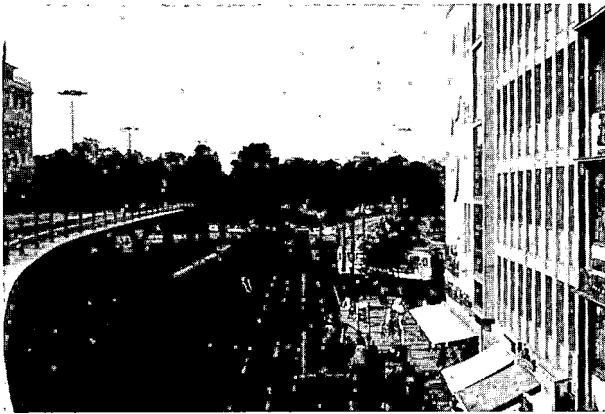
P-51. A 4-track light rail facility with stops in a pedestrian area. Highway viaduct on left (Düsseldorf)
