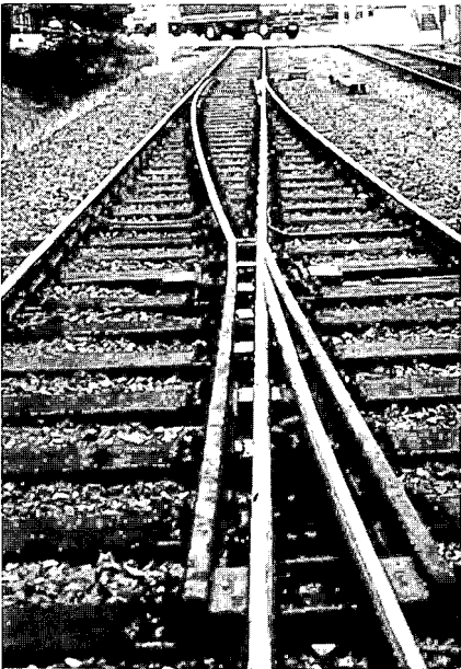
P-48. The latest type of switch: frog also has an elastic point. Straight position
