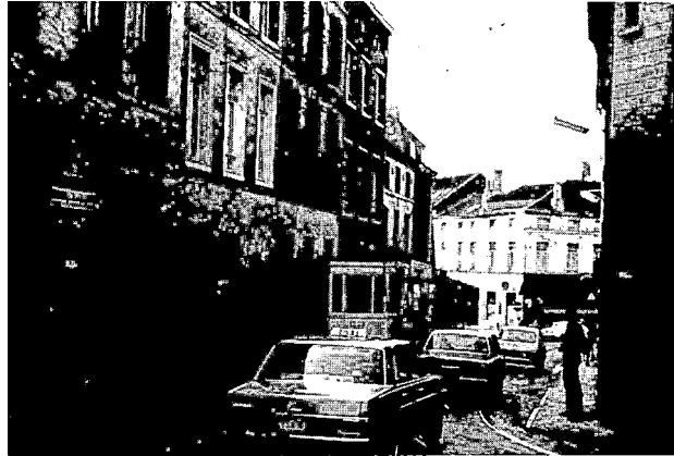
P-21. Old type streetcar operation: slow and unreliable (Brussels)
