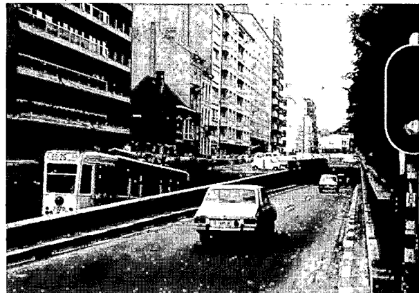
P-46. Tunnel access ramp (Brussels)
