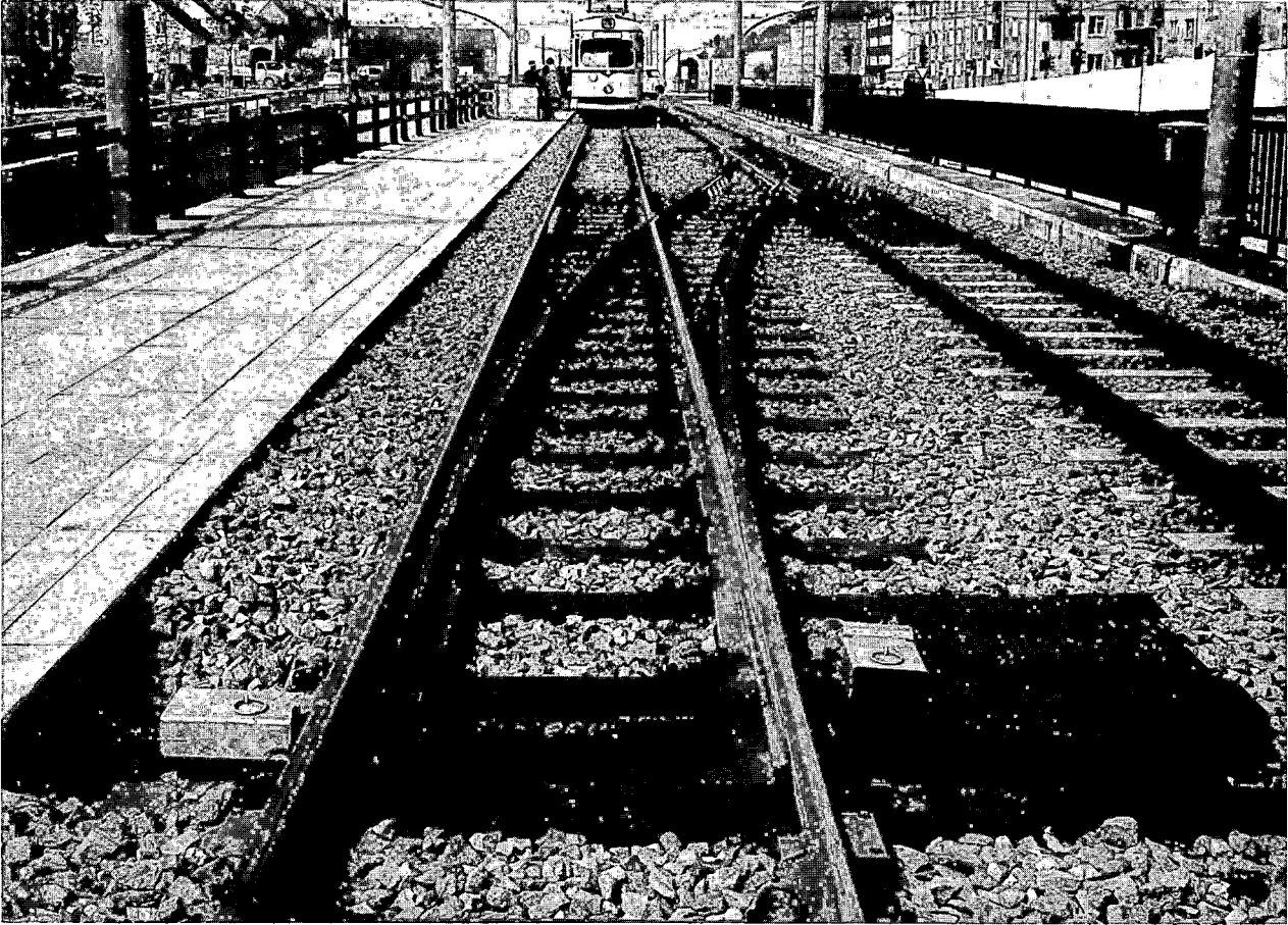
P-47. Modern switch with elastic points
