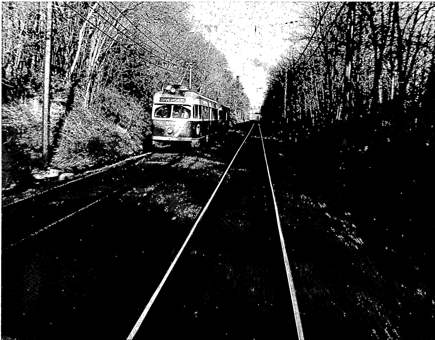
Figure 1-2 Typical Green Line Right of Way
