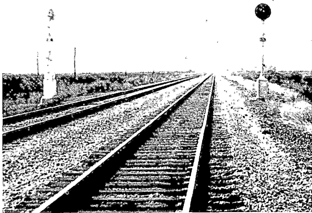
Fig. 6. Illustration of test site—freight car truck development—test track section, high speed running, main line west, Suisun, Ca., MP-43.3.
