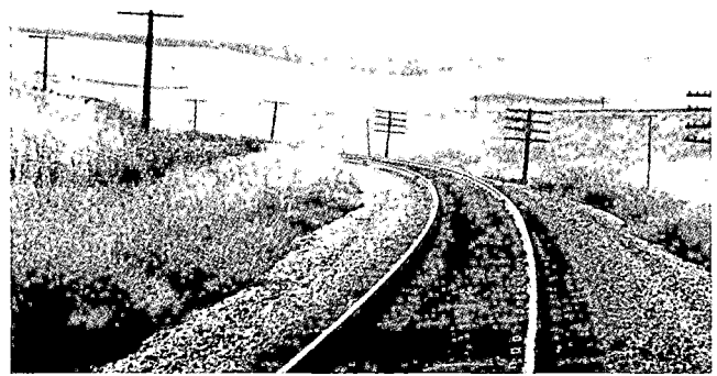
Fig. 8. Illustration of test site—freight car truck development—test track section, curve negotiation, 1% grade, Altamont-Ulmar, Ca., MP-53.
