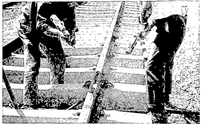
Fig. 6. B-66 ties with Pandrol fasteners at Noble, Illinois.
