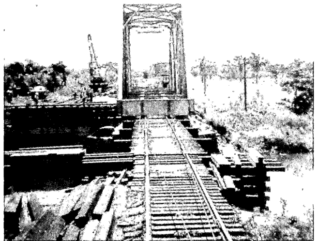
Fig. 24. Juanita River Bridge.
