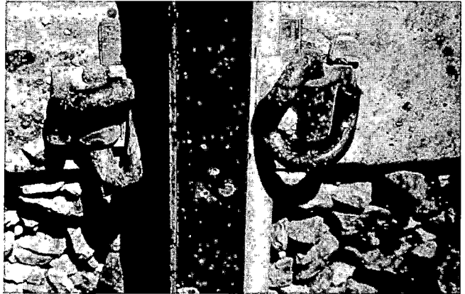
Fig. 9. British Costain concrete tie and pandrol 607-A fasteners at Lorraine, Virginia.
