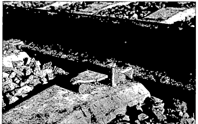
Fig. 10. Gerwick RT -7S concrete ties and British trec CS-5 fasteners at Lorraine, Virginia.
