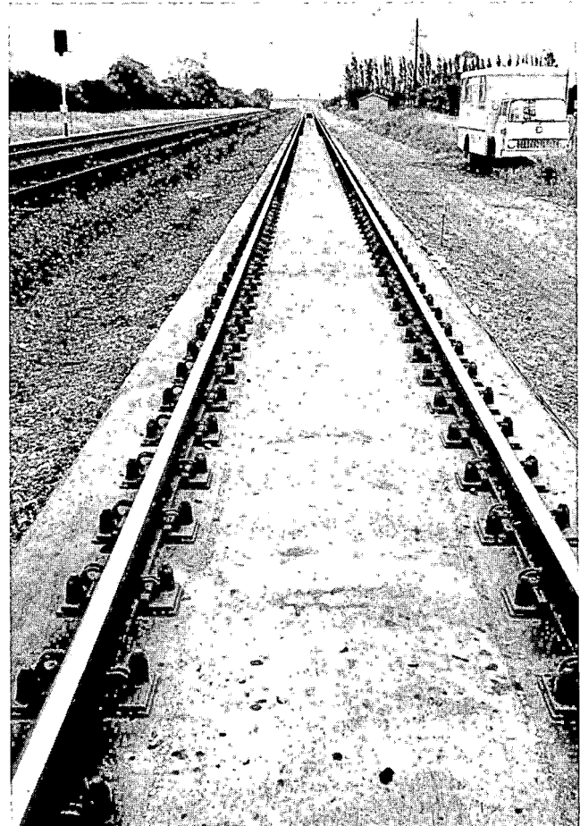
Fig. 9. Radcliffe test slab track.
