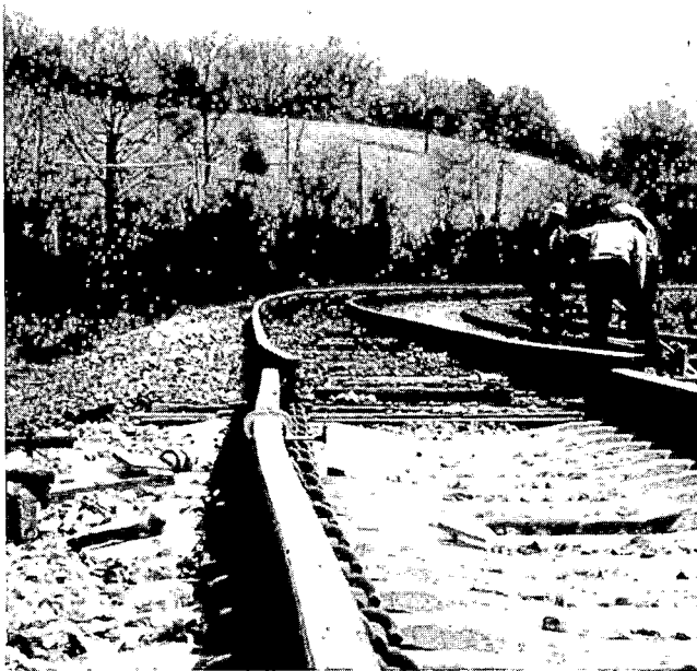
Fig. 18. Displaced concrete tie panel.
