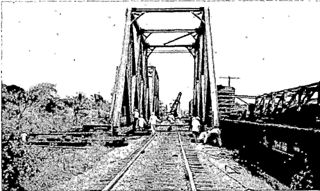
Fig. 8. New trusses for bridge over Cotaxtla River.
