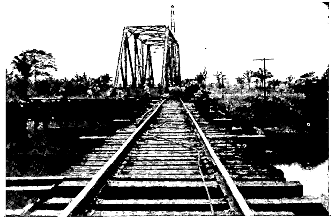
Fig. 22. Juanita River pulling the new truss over the old bridge.
