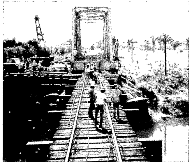
Fig. 23. Juanita River Bridge installation of the new truss.
