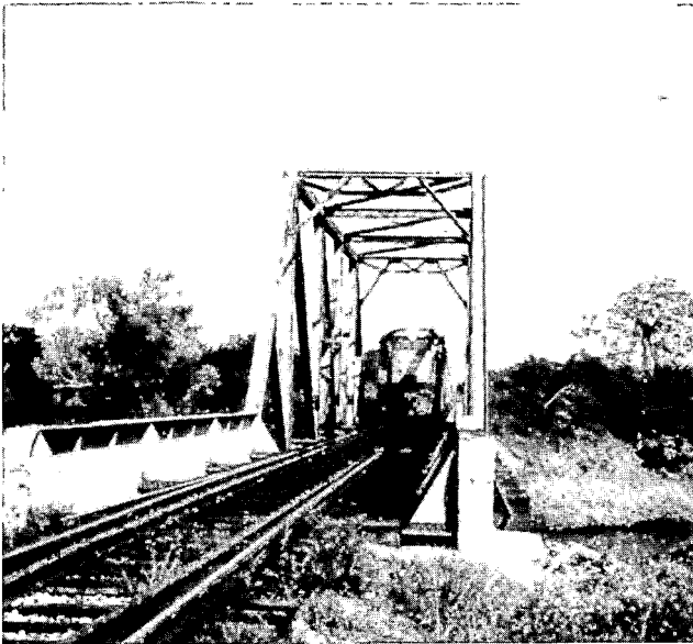
Fig. 19. Juanita River Bridge installation of the new truss.
