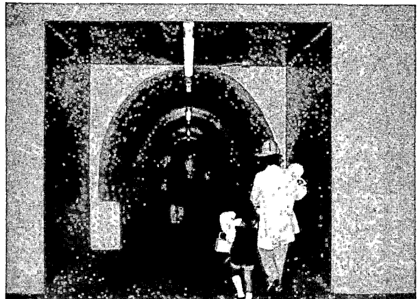
8. Tunnel Leading to Stairs to Westbound Platform
