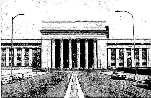
1. Main Entrance on West Side of Terminal
