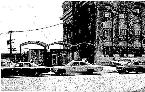
1. Canopy Entrance to Existing Terminal
