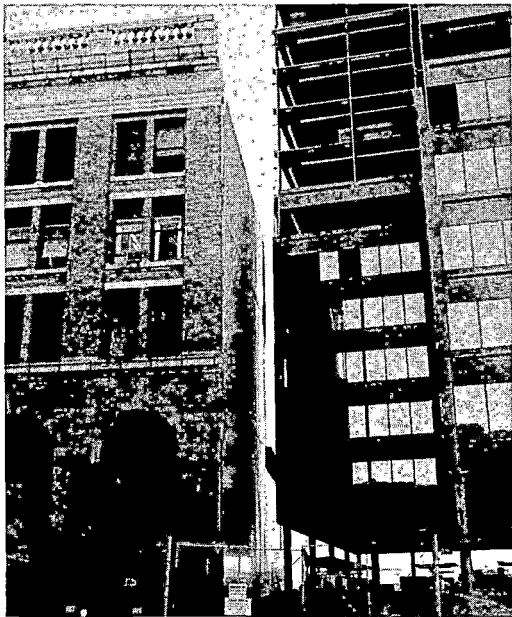
5. Adjacent Office Building Showing Temporary Closure Wall in Terminal
