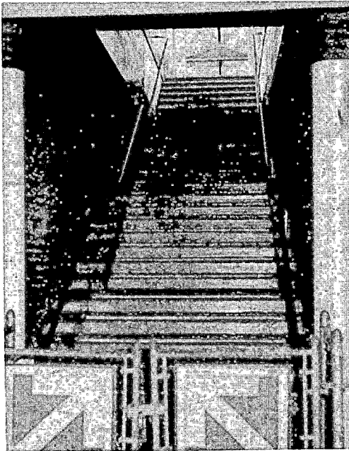
7. Gated Stairway to Center Platform
