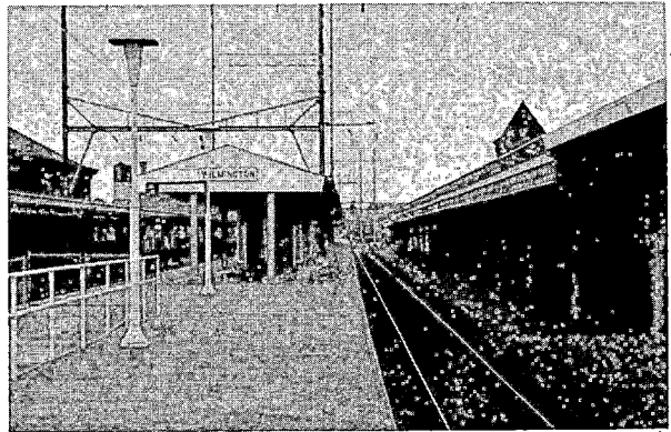
6. Terminal Platform Level and Waiting Area
