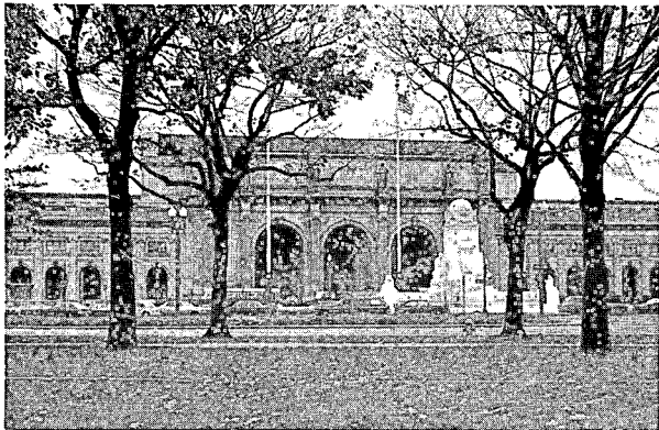
1. Main Entrance Facade and Covered Porticos
