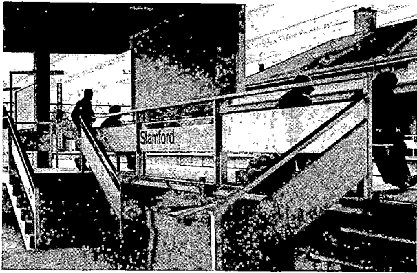
3. Canopied Stairways to Platforms
