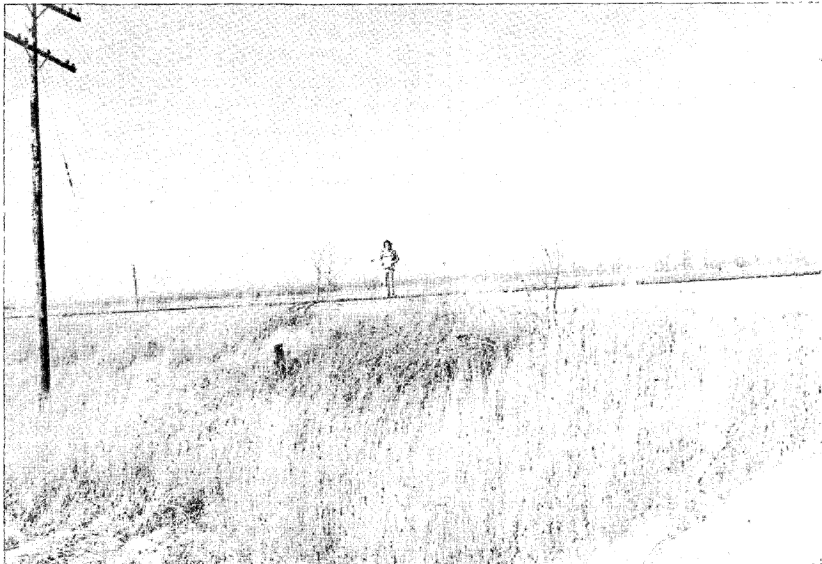
Embankment Near Ark. Highway 149 Crossing
