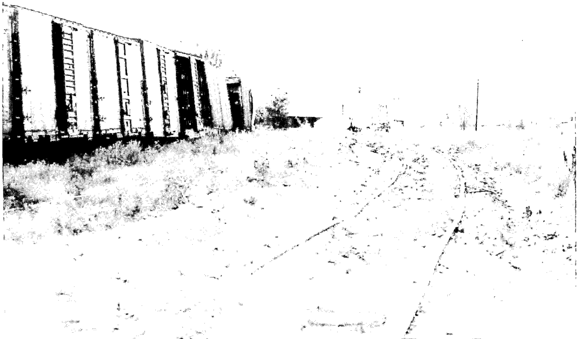
Bentonite Spur Roadbed Shortly After Injection
