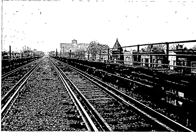
TYPICAL VIEW OF BALLASTED DECK OF ELEVATED STRUCTURE.
