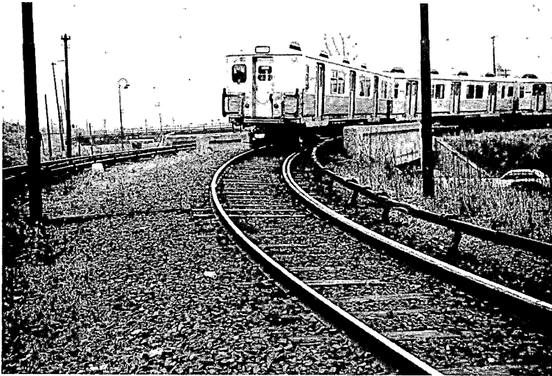
THE TEST SECTION IS IN THE FOREGROUND
