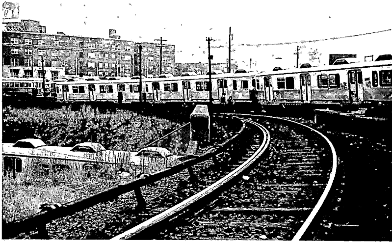
TRANSITION BETWEEN TEST SECTION AND CONTROL SECTION OCCURS AT BRIDGE. THE CONTROL SECTION IS IN THE FOREGROUND.
