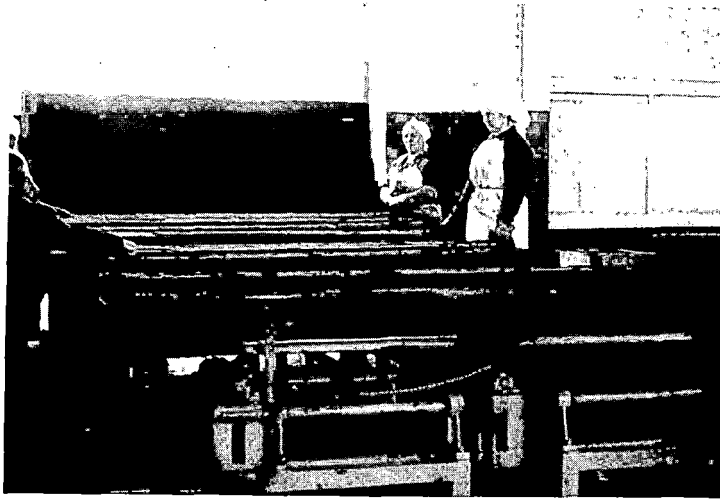
FIGURE 8.7 VISUAL INSPECTION OF TIES ENTERING PLANT
