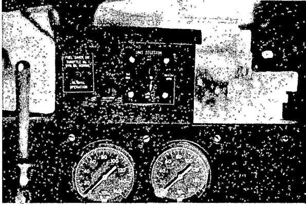
FIGURE 1. FUEL SAVER CONTROL BOX ON LOCOMOTIVE CONTROL STAND
