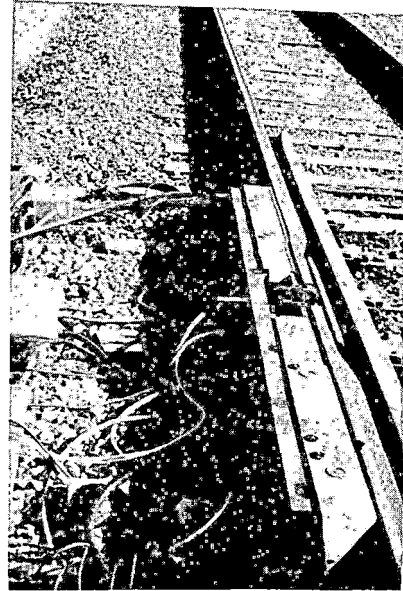
FIGURE 61. WAYSIDE INSPECTION COMPONENTS
