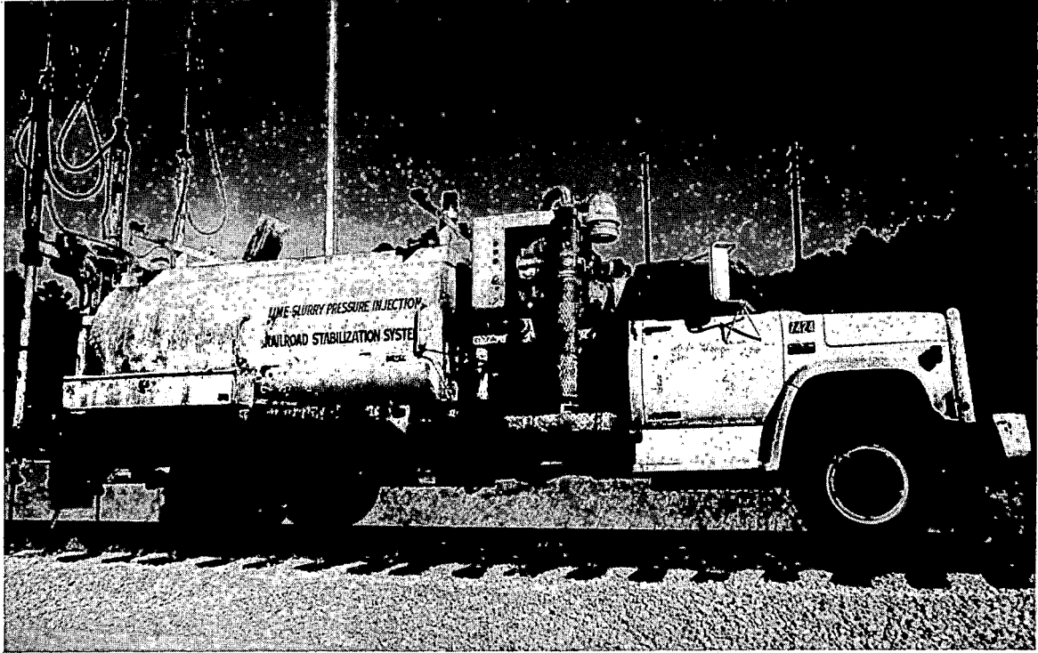
Fig. 2. Lime injection truck.
