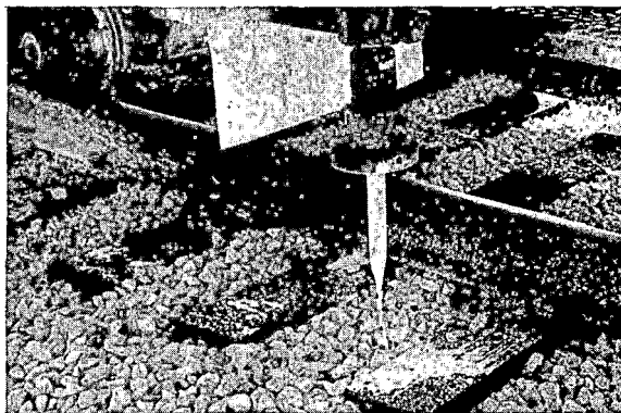
Fig. 7. Lime injection nozzle.
