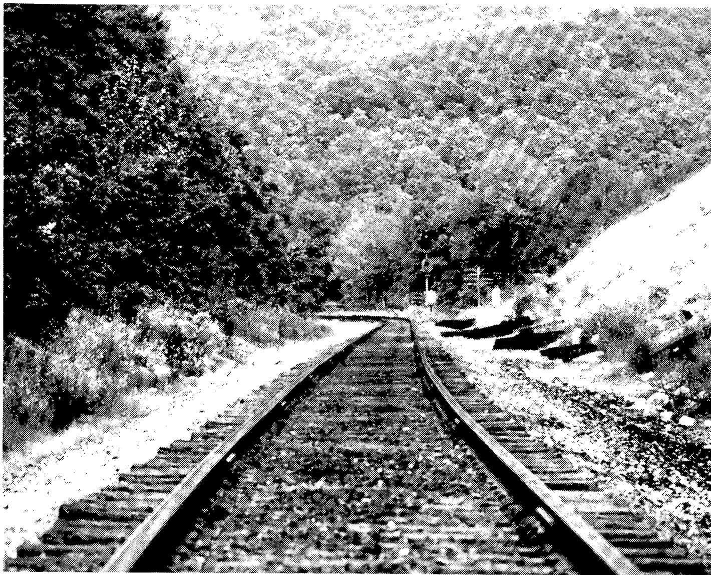
FIGURE 3-6 PARTIAL VIEW OF TEST ZONE
