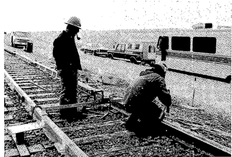
177. TRACK REBUILD - FINAL ADJUSTMENTS
