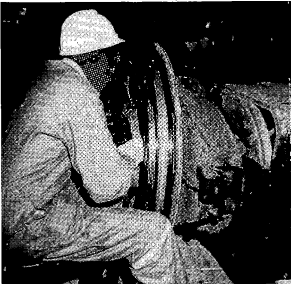
127. REMOVING WATERPROOF/PROTECTIVE COATING TO EXPOSE STRAIN GAGES ALSO SHOWING TRACTION MOTOR
