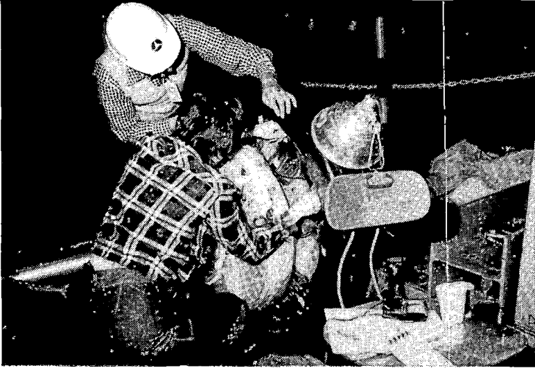
149. INSTALLING NEW WIRES
