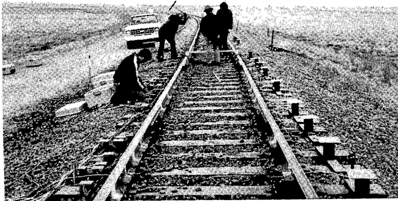
176. TRACK REBUILD - RESPIKING LOW RAIL
