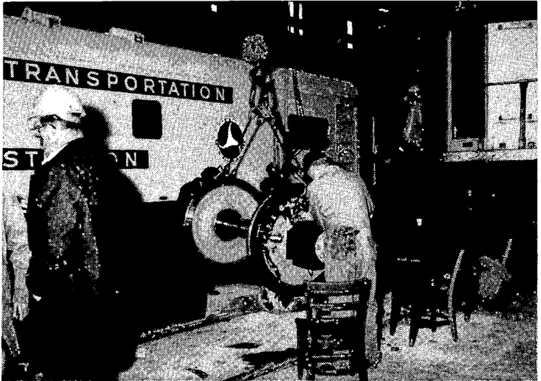
130. HOISTING DAMAGED WHEELSET TO NEW WORKING LOCATION
