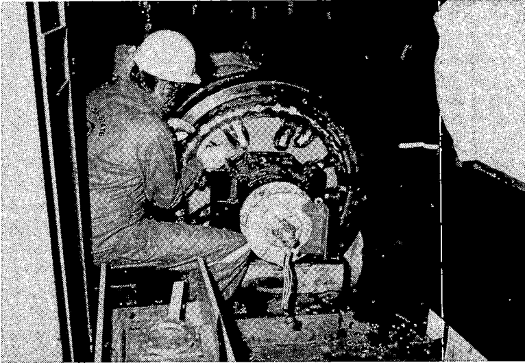
141. REMOVING PROTECTIVE COATING TO EXPOSE JUNCTION BOARD
