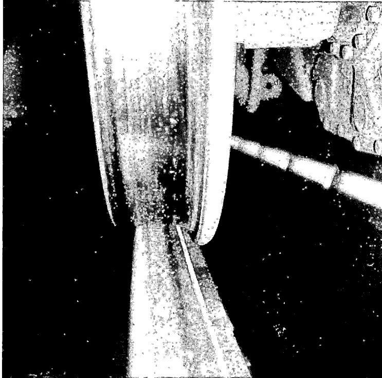
FIGURE 10-1. TYPICAL WORN WHEEL IN ATLANTA.
