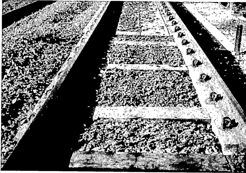
FIGURE 3-50. TRANSITION BETWEEN SLAB TRACK AND BALLASTED TRACK
