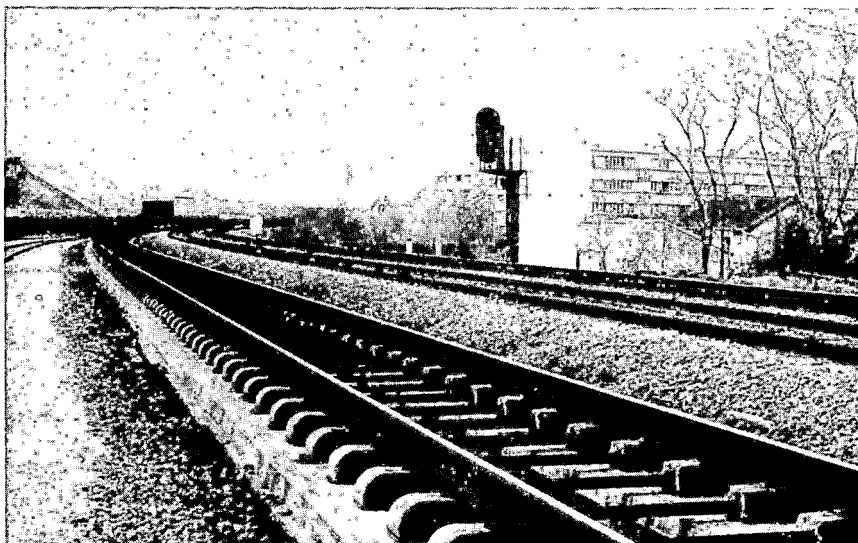
FIGURE 3-46. SLAB TRACK AT NEUILLY-SUR-MARNE
