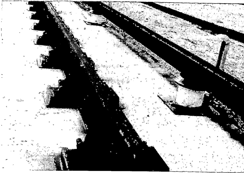
FIGURE 5-13. THIRD RAIL CHAIR ASSEMBLY SECURED TO SLAB
