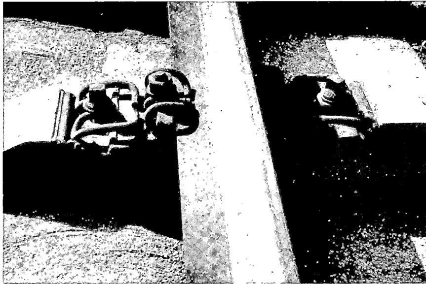
FIGURE 4-10. GERMAN RAILWAYS FASTENER AT KARLSFELD
