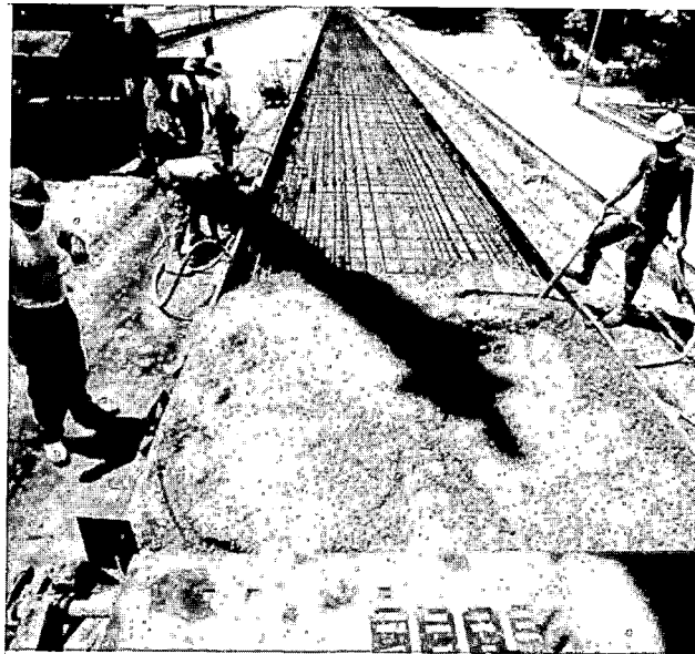
FIGURE 5-4. CONCRETE PLACEMENT AND CONSOLIDATION
