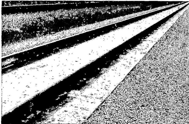
FIGURE 3-57. SLAB TRACK ON THE KANSAS TEST TRACK
