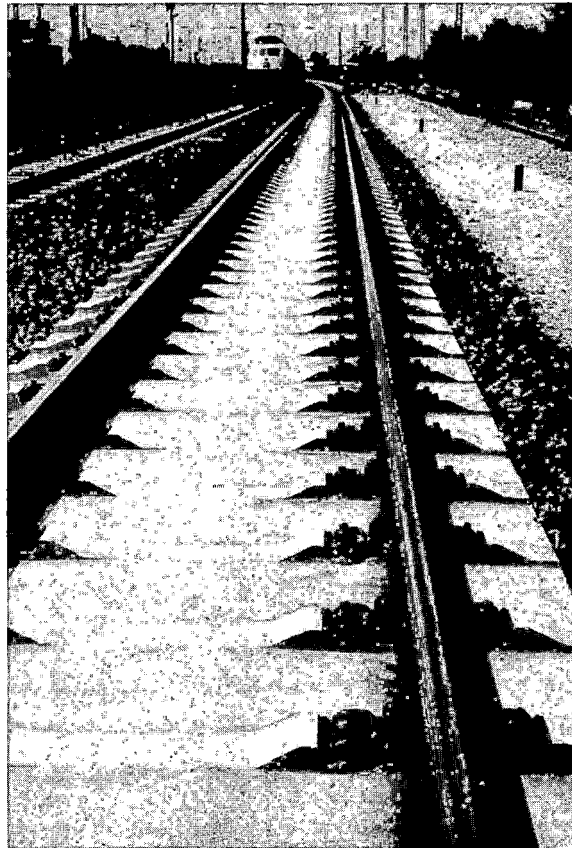
FIGURE 3-27. SLAB TRACK AT RHEDA
