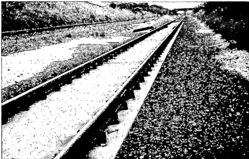
FIGURE 3-18. PRECAST CONCRETE SLABS AT RADCLIFFE-ON-TRENT
