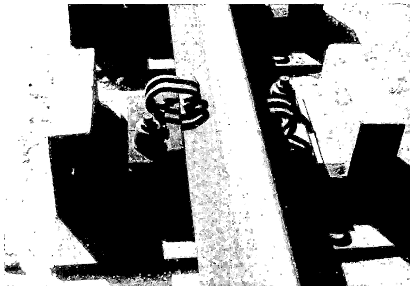
FIGURE 4-12. NETHERLANDS RAILWAY FASTENER AT KARLSFELD-TYPE 1
