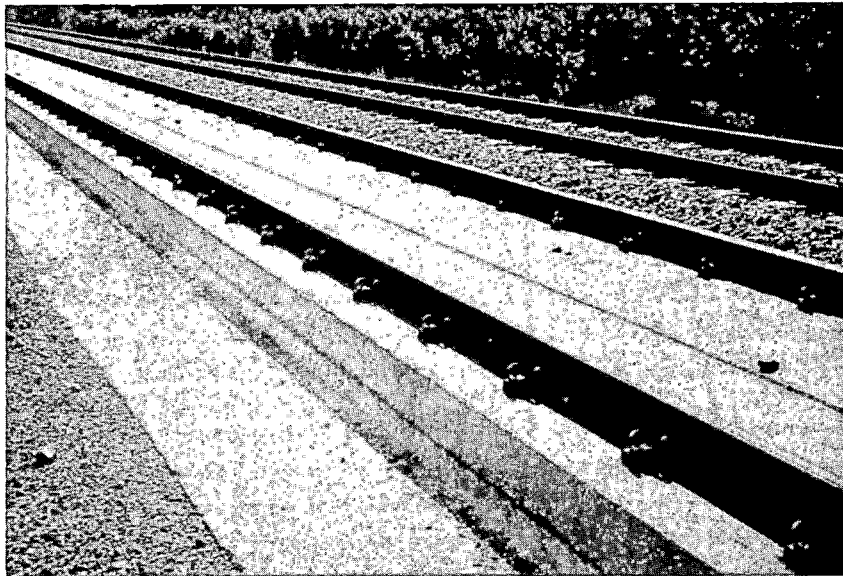
FIGURE 3-48. SLAB TRACK BETWEEN RICLA AND CLATORAO
