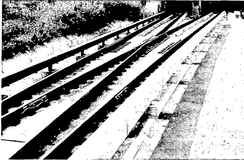
FIGURE 3-56. TURNOUT ON SLAB ON METROPOLITAN ATLANTA RAPID TRANSIT AUTHORITY
