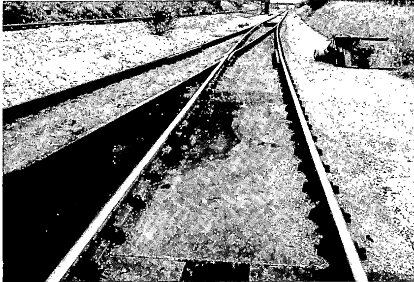
FIGURE 3-15. TURNOUT ON SLAB AT RADCLIFFE-ON-TRENT
