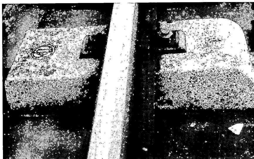
FIGURE 4-3. SWISS RAILWAYS FASTENER AT RADCLIFFE-ON-TRENT
