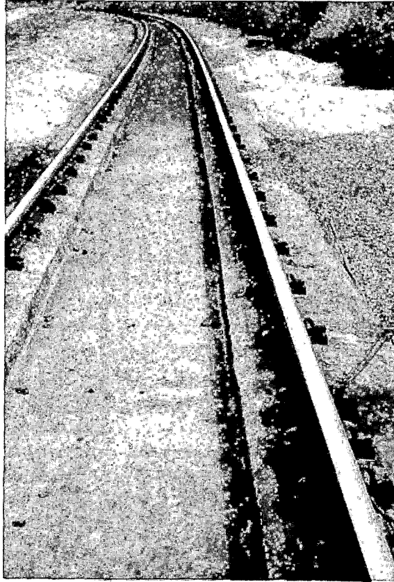
FIGURE 3-13. BRITISH RAILWAYS DIRECT-LAID TRACK AT RADCLIFFE-ON-TRENT
