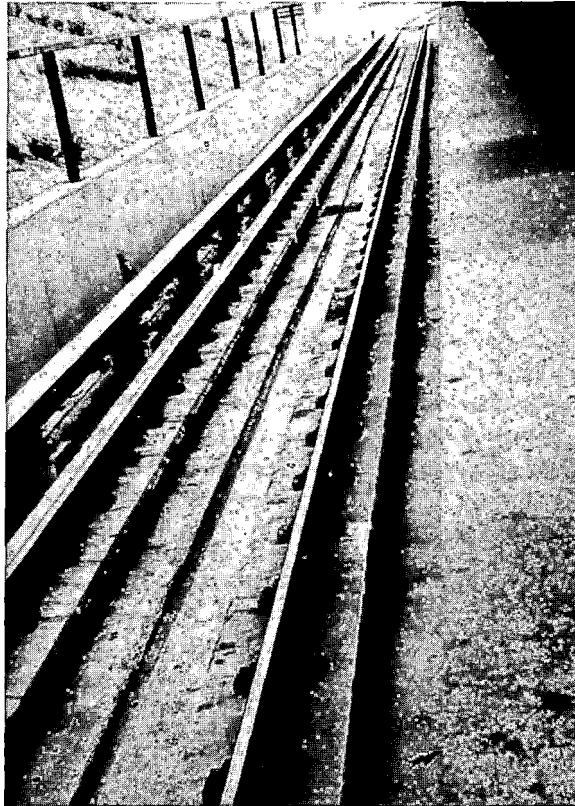
FIGURE 3-54. SLAB TRACK ON METROPOLITAN ATLANTA RAPID TRANSIT AUTHORITY
