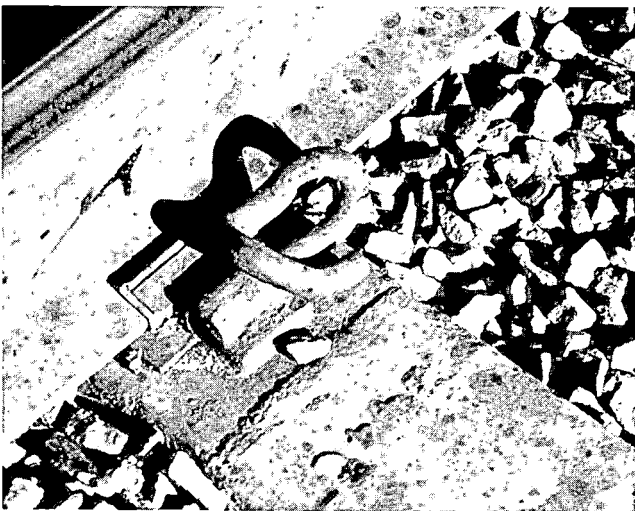
FIGURE 6. CLIP FALLOUT, PANDROL CLIP.
