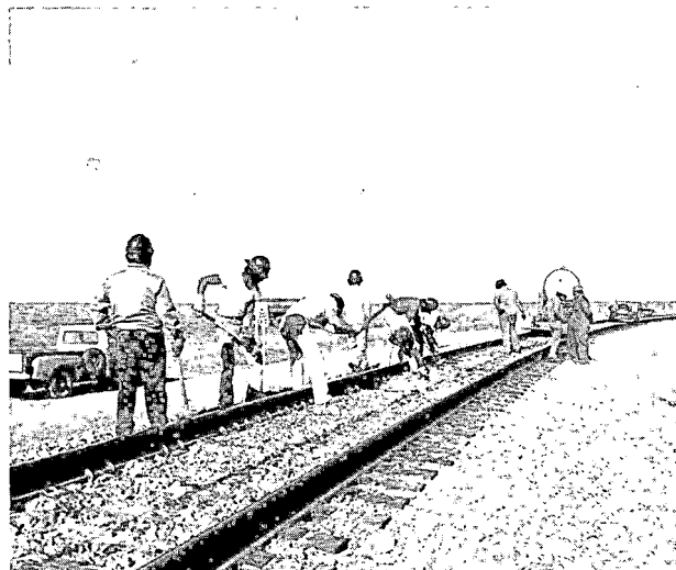
FIGURE 5. TRACK REBUILD.
