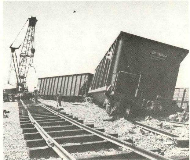
FIGURE 2. THE RESULTS OF INADEQUATE TRACK MAINTENANCE.
