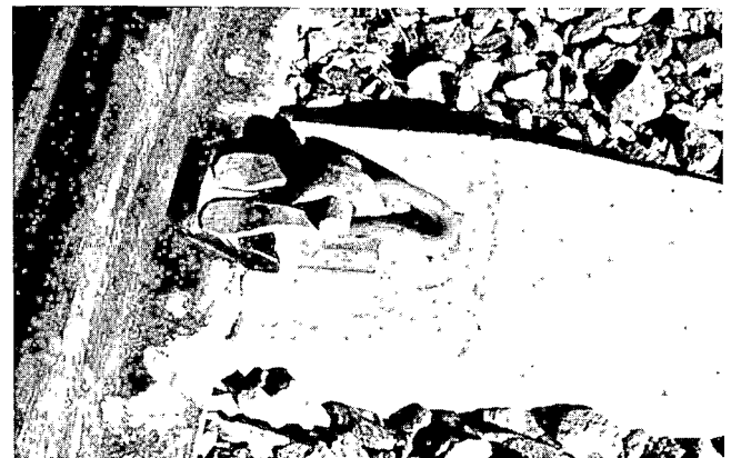
FIGURE 15. VSD FASTENER SYSTEM.
