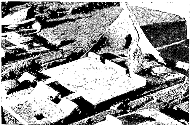
FIGURE 7. TIE PAD EXTRUSION SECTION 2 AT 359 MGT.
