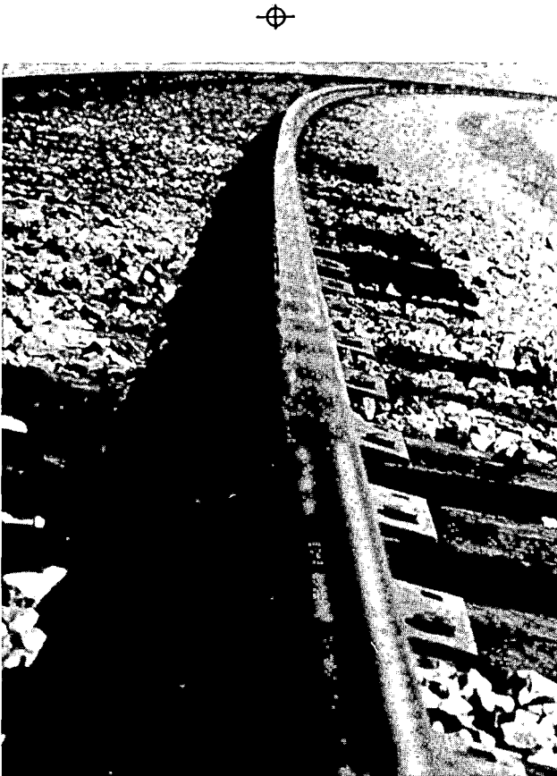
FIGURE 1. LOW RAIL CORRUGATIONS AT SECTION 3, 5° CURVE, 73 MGT.
