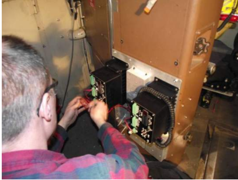
Figure 16. Wiring the Control Panel (ANC controller on left and AVC controller on right)
