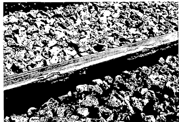
FIG. 9: TYPICAL SHELL DEFECT
