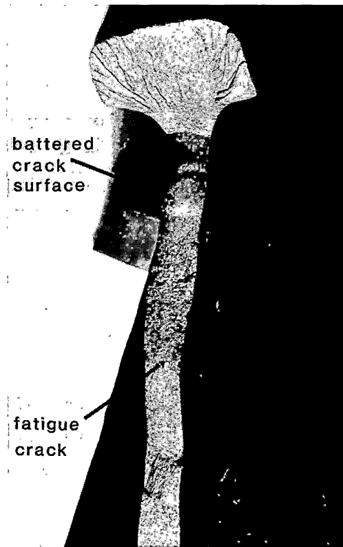
FIGURE 51. THERMITE WELD FAILURE.
