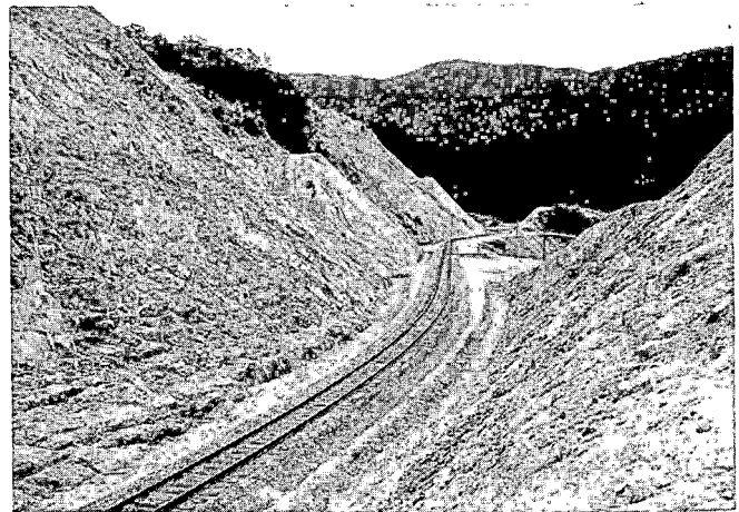
Photo. No. 9. Goonyella Line.
