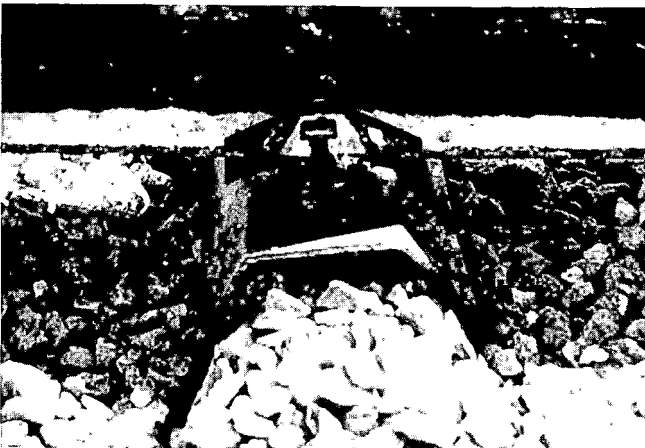
Fig. 4 Ballast Under Sleeper After One Tamp
