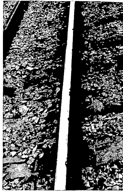
Fig. 9 Multiple "light" shelling on a rail length.
