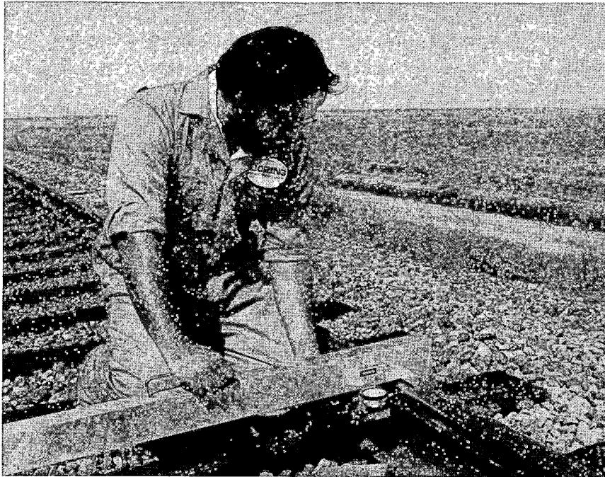
Track Gage Measurement on FAST Track
