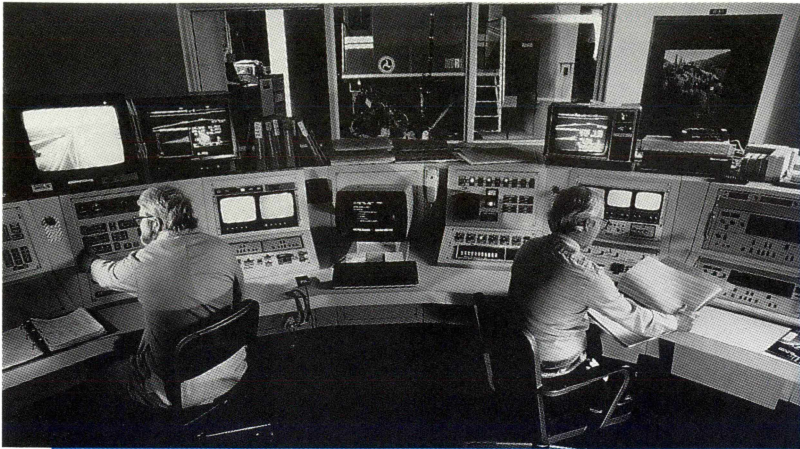
Trainers set up operating conditions and monitor student performance from a remote operating console. This photo shows the RALES facility, a full-function locomotive simulator located at IITRI's Chicago headquarters.
