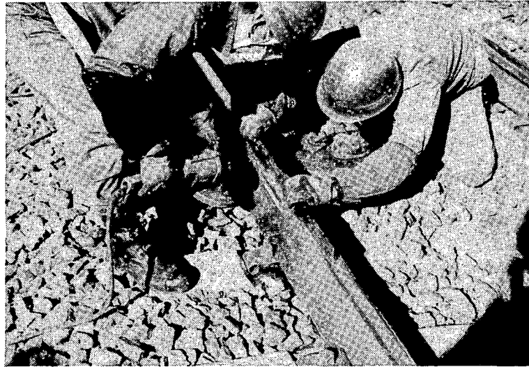
Fig.31 Final Grinding for Meeting Track Geometry Standard
