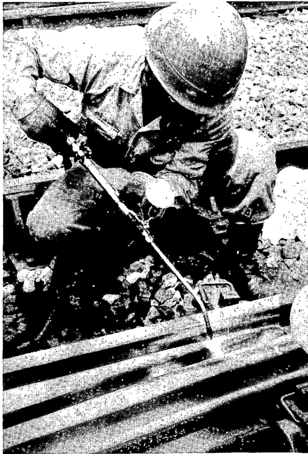
Fig.33 Gas Spray Welding for Nose Rail of Welded Crossing
