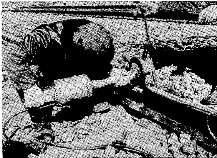
Fig.26 Grinding of Engine Burn
