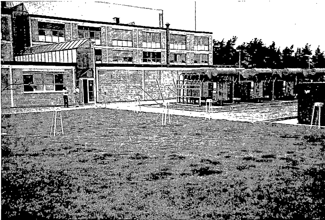
FIGURE 25A TRANSFORMER YARD PROFILE LOOKING NW (INVERTER BLDG. AND CONTROL CENTER IN BACKGROUND)
