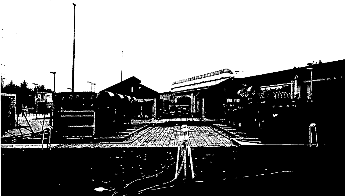
FIGURE 25B TRANSFORMER YARD, LOOKING NORTH. BRAKING RESISTOR BANKS IN SHELTERS BEHIND TRX YARD
