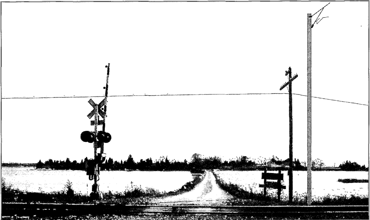
FIGURE 4.11-12(a). COMPARISON OF THE HISTORIC POLE LINE AND THE FUTURE CATENARY SYSTEM LOOKING SOUTH AT FREEMAN'S CROSSING, STONINGTON, CT
